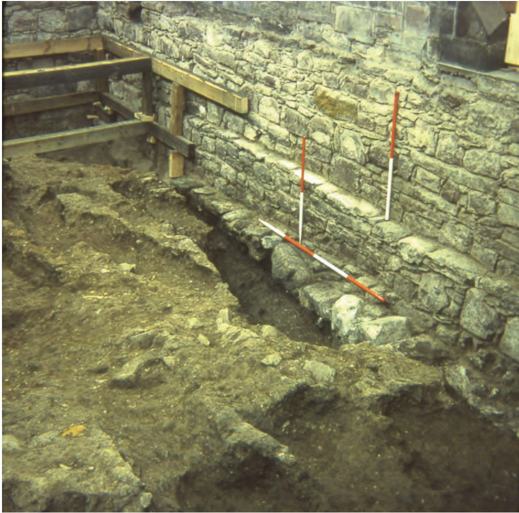
Illus 23 Underpinning of south wall in Period 3b
