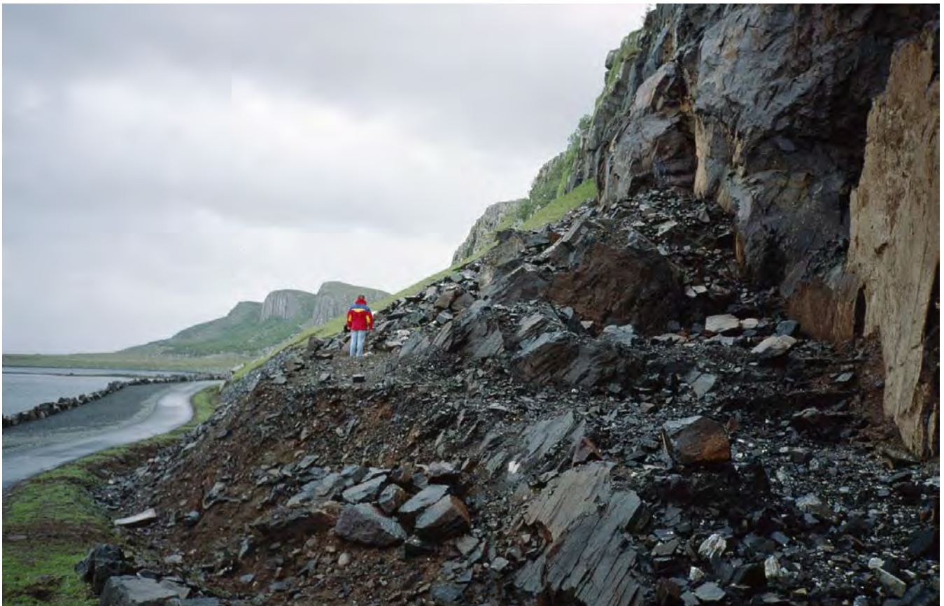
Illus 11 Situation in June 1994 subsequent to the rockface blasting, viewed from the north (photo: Alan Saville)
