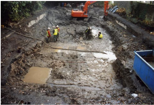
Illus 18 View of timber piles and Trench 2, looking south
