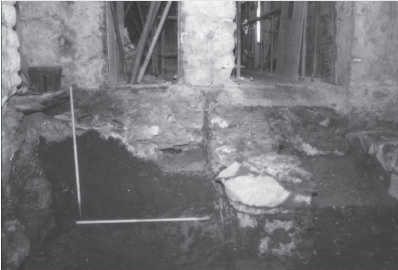
Figure 3.12 Wall of a tenement building surviving under Queensberry House
