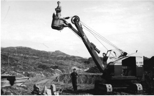
Illus 4 Utilizing quarry machinery as a photographic platform (pre-Health and Safety days!)
