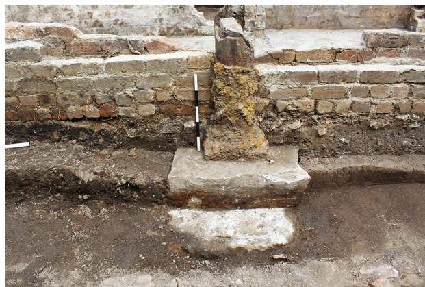
Illus 18 Example of hollow cast iron columns
