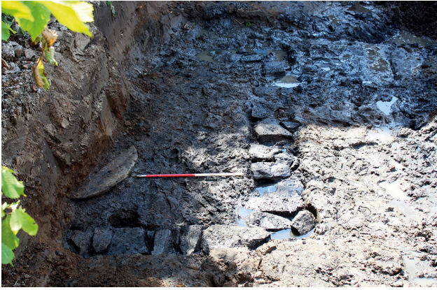
Illus 12 Stone Structure [276], looking south-west
