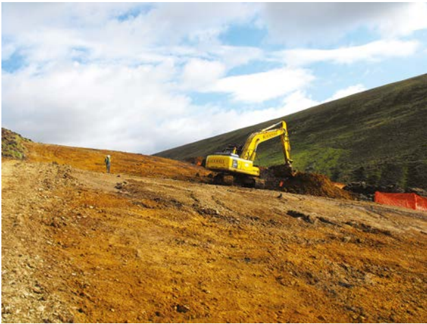
Illus 5.2 Monitoring topsoil stripping for access track on southern slopes of Midlock Valley. (© Headland Archaeology (UK) Ltd)
