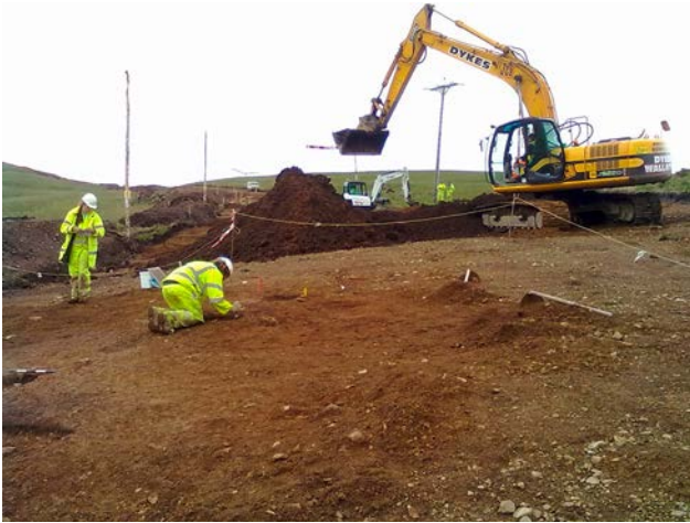
Illus 2.3 View south of topsoil stripping for access road on southern side of Midlock Valley. (© Headland Archaeology (UK) Ltd)
