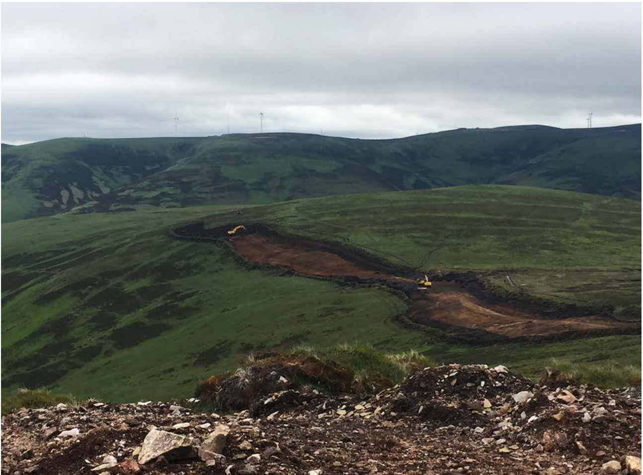
Illus 7.7 Excavating access road Zone 3. (© Headland Archaeology (UK) Ltd)
