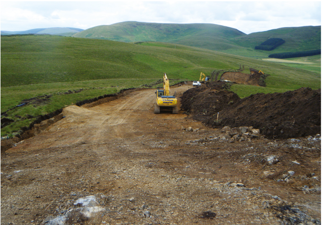
Illus 4.1 View west of topsoil stripping for access road on the southern side of Camps Valley. (© Headland Archaeology (UK) Ltd)
