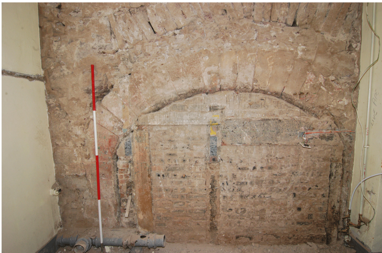
Illus 31 The G12 fireplace showing the segmented arch of the 16th-century fireplace with a later blocked fireplace and coal cupboard. (© CFA Archaeology Ltd)
