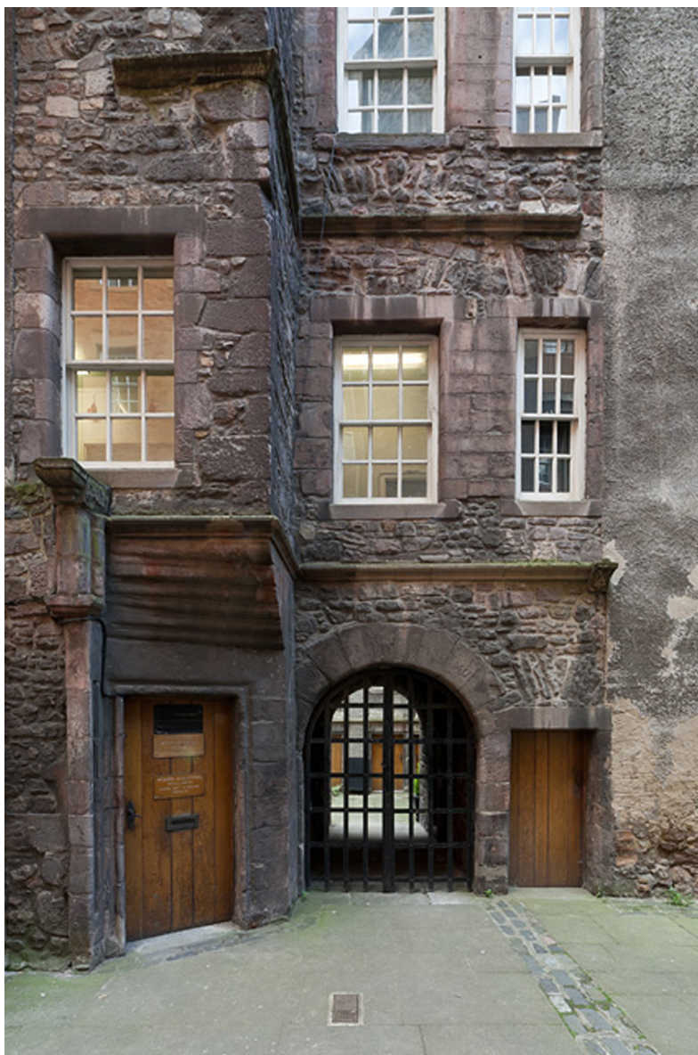
Illus 23 External north-facing elevation. (© Scottish Historic Buildings Trust)
