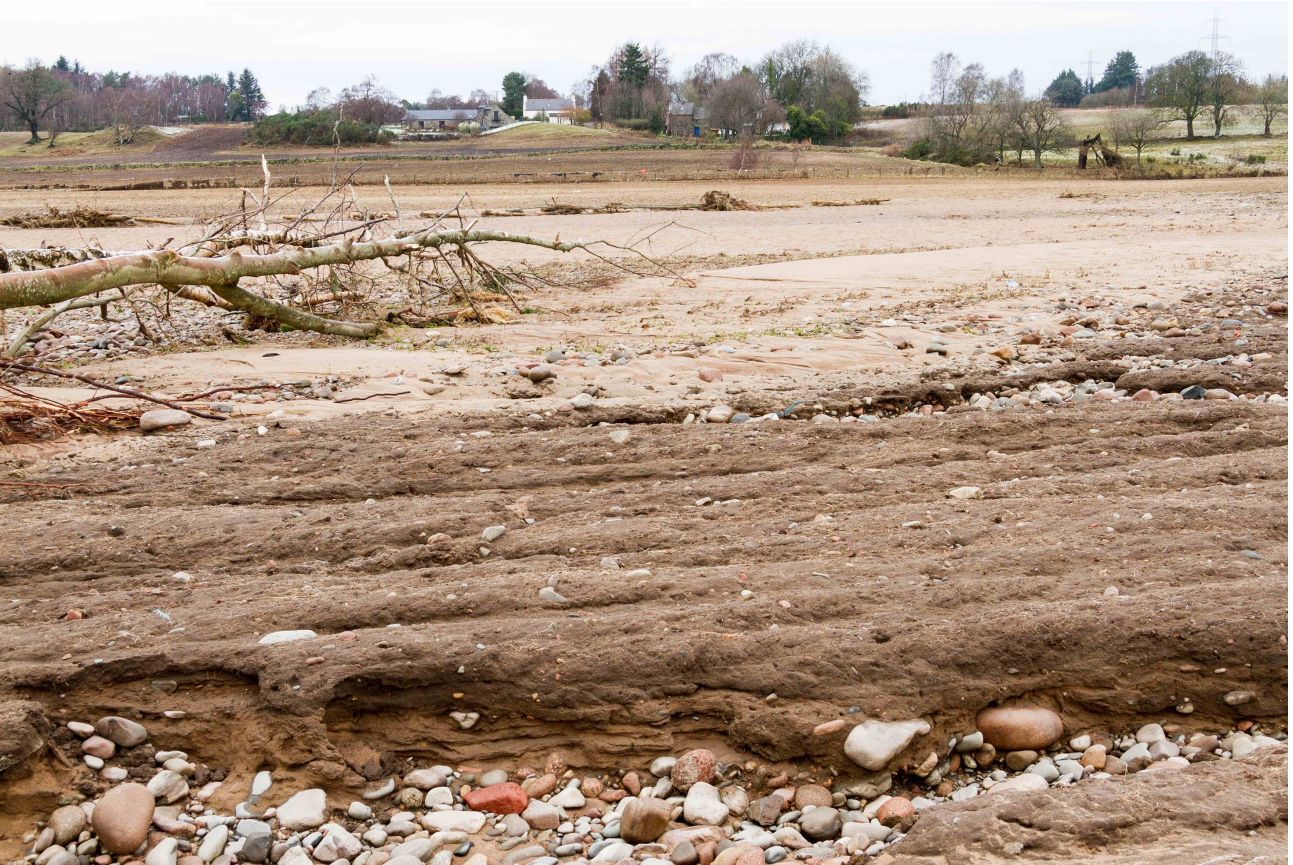
Illus 4.3 Damage caused in 2015 by Storm Frank, looking north across field NM5 to the houses at Mills of Drum. Note the fallen tree, veneer of fresh sand and eroded plough furrows
