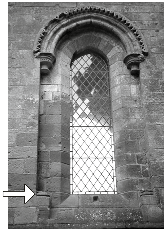
Illus 13 Example of shaft base as seen in a window at Dryburgh Abbey © Richard Fawcett
