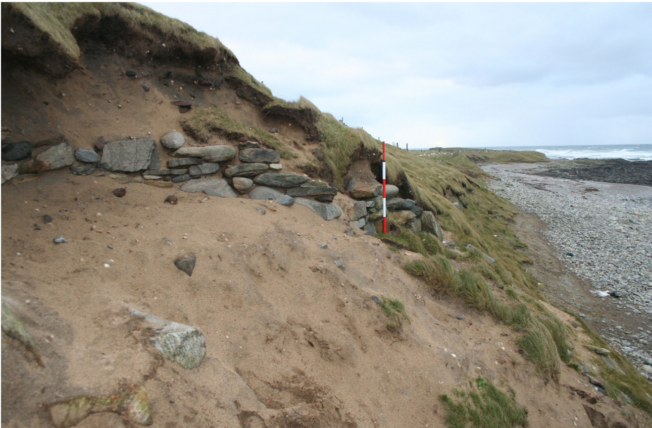
Illus 14 Cliff line north of the graveyard at South Galson showing eroding structures
