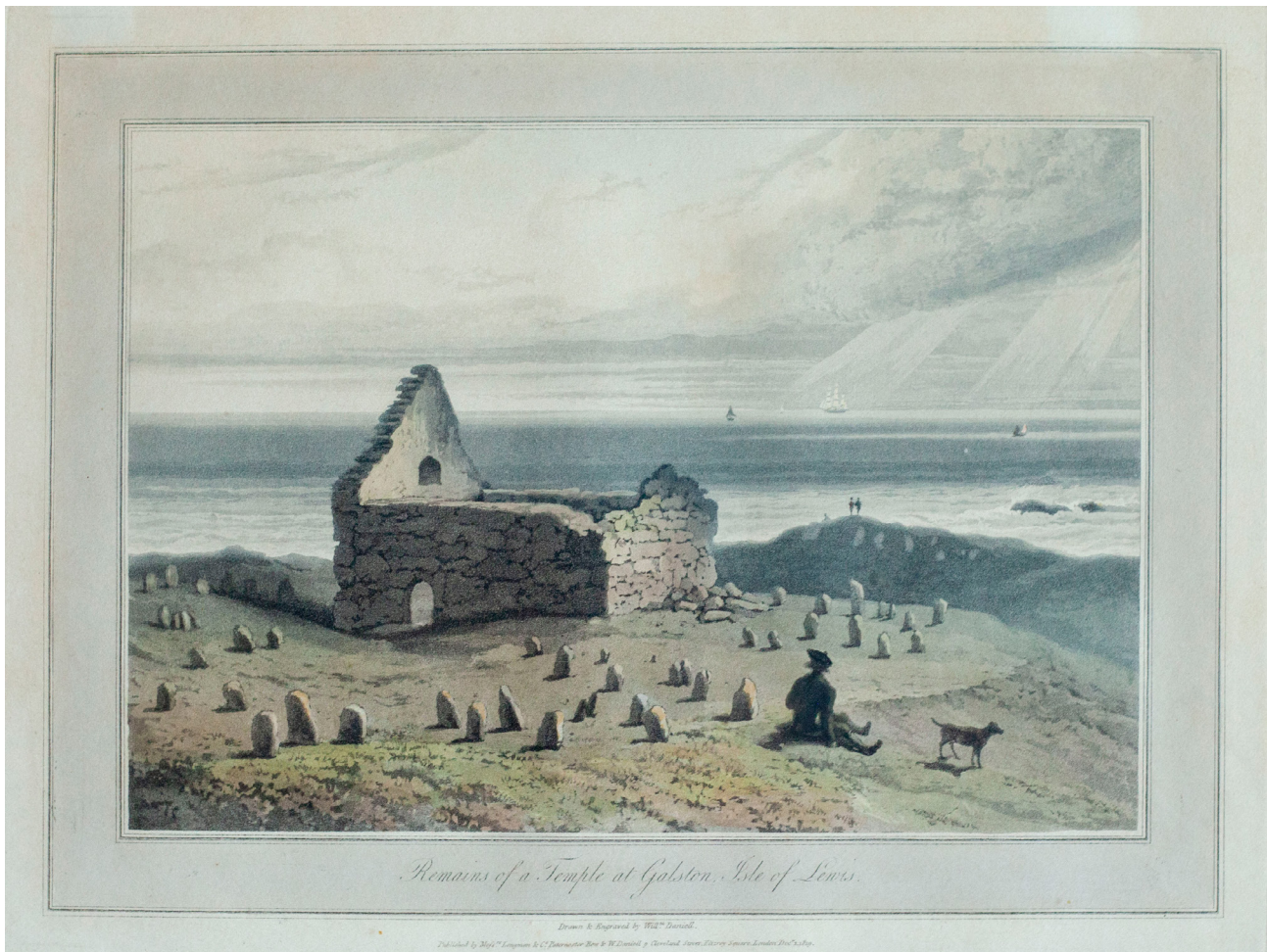
Illus 12 William Daniell's engraving (1819) of 'Remains of a Temple at Galston, Isle of Lewis' (reproduced by Fiona Rennie from an original print by kind permission of Agnes Rennie, South Galson)
