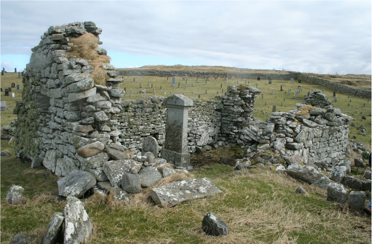
Illus 36 North-west corner of nave and entrance in the south wall, from the south-west
