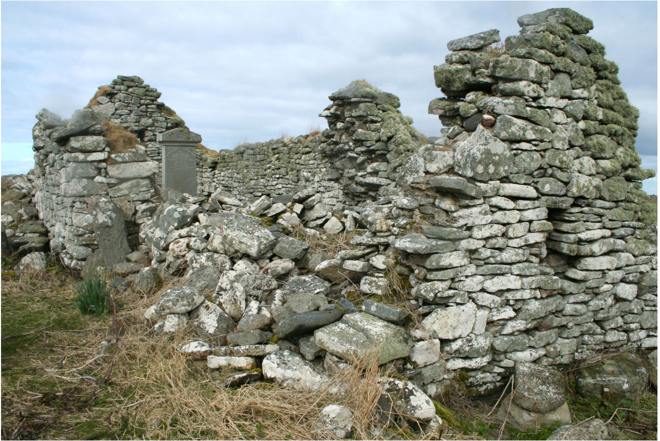
Illus 38 Detail of collapsed south wall of chancel from the south-east
