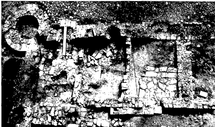
ILLUS 14 Phase 5: Structure E, in the south barmkin; modifications include subdivision of the west room, paving and a doorway opening onto the cobbled outer yard (Structure H)
