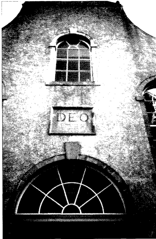
ILLUS 5 Classical façade of the late 18th-century Catholic church of St Gregory's, Preshome: 'Deo 1788'
