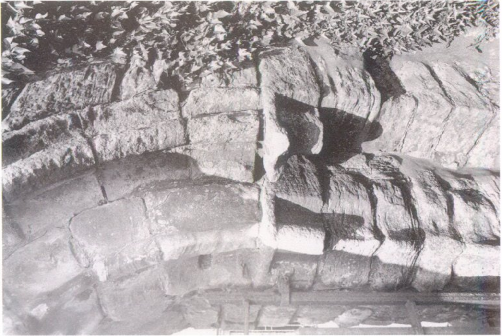
ILLUS 24 St Cuthbert, Monkton: detail of east jamb of south portal
