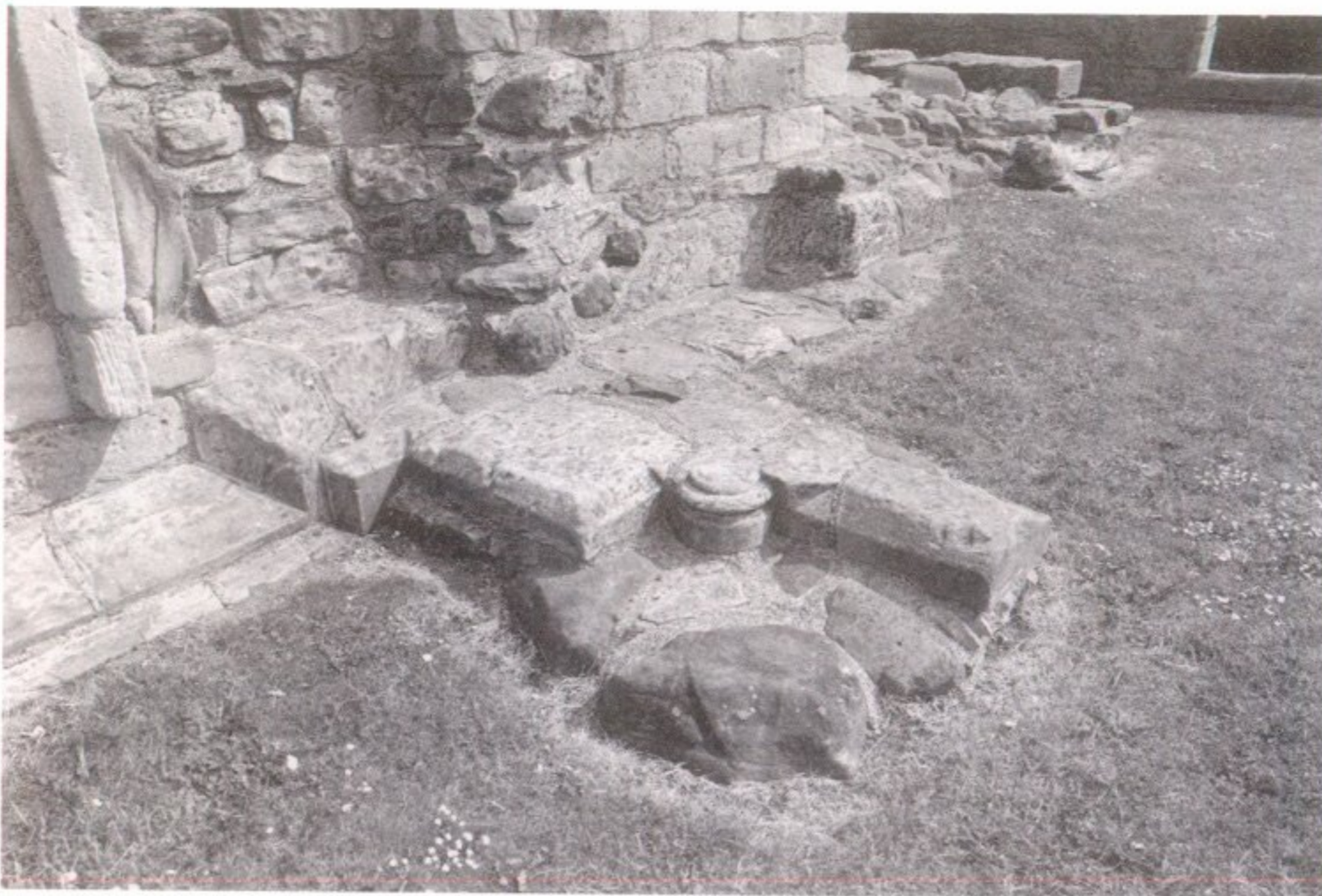
ILLUS 47 Remains of intended new west wall of west range with base for jamb shaft of portal
