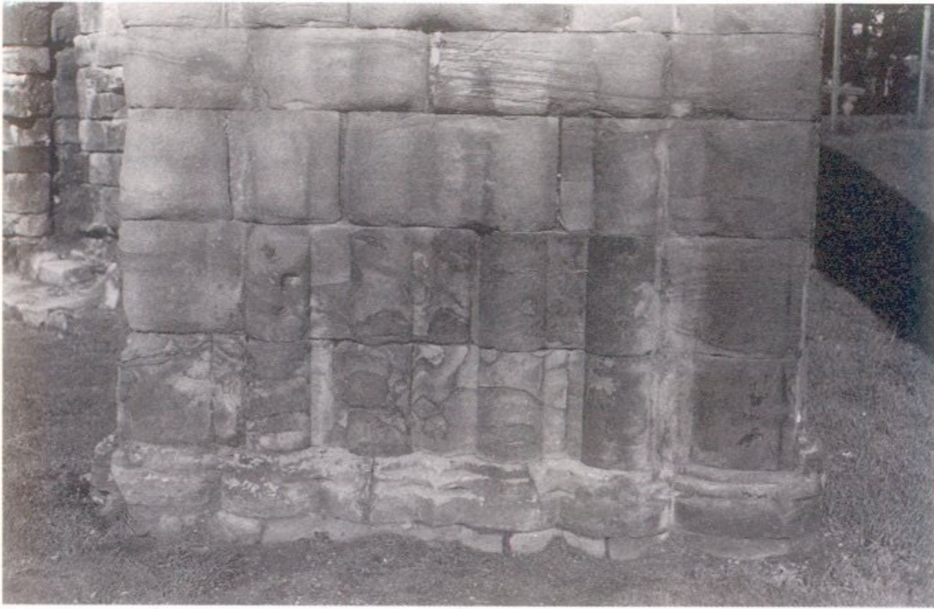
ILLUS 41 Base of pier at end of south nave aisle
