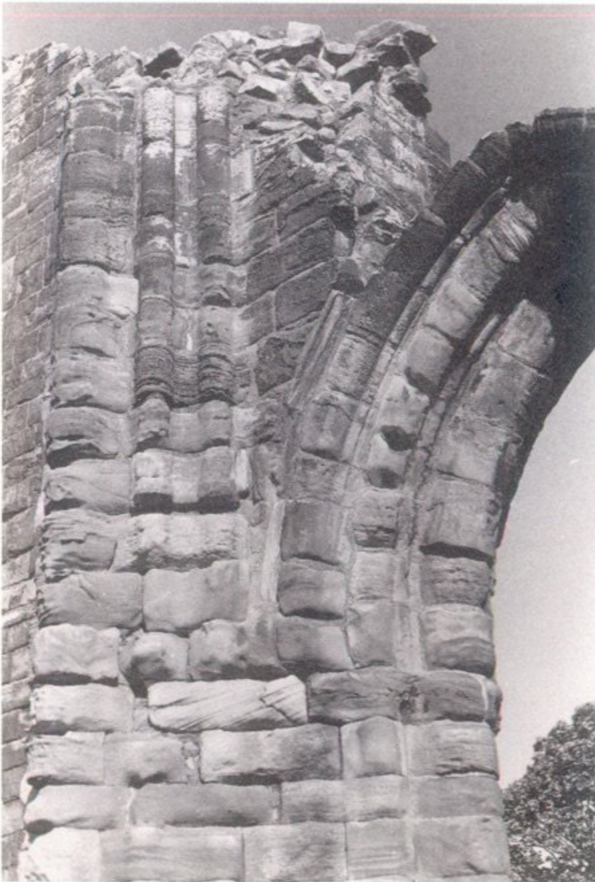
ILLUS 42 Detail of pier and arch at end of south nave aisle
