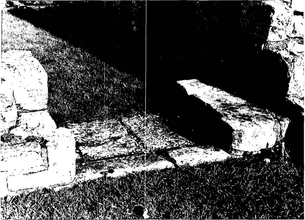
ILLUS 22 Threshold of portal at south end of west range
