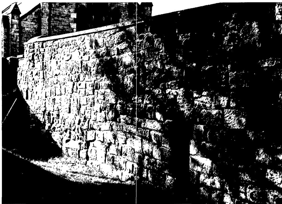
ILLUS 20 Exterior face of east wall of east range
