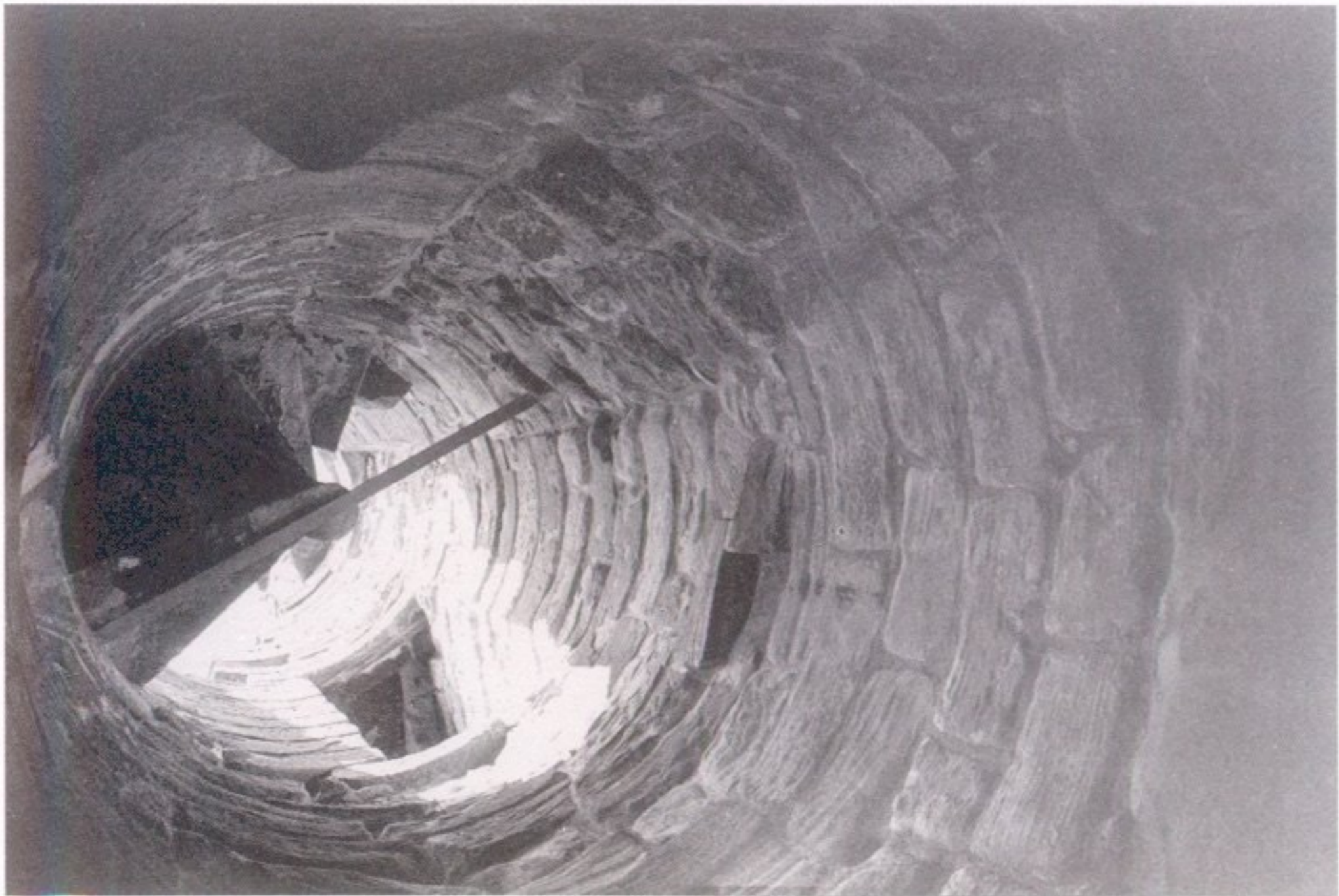
ILLUS 39 View of newel stair in south-west angle of transept
