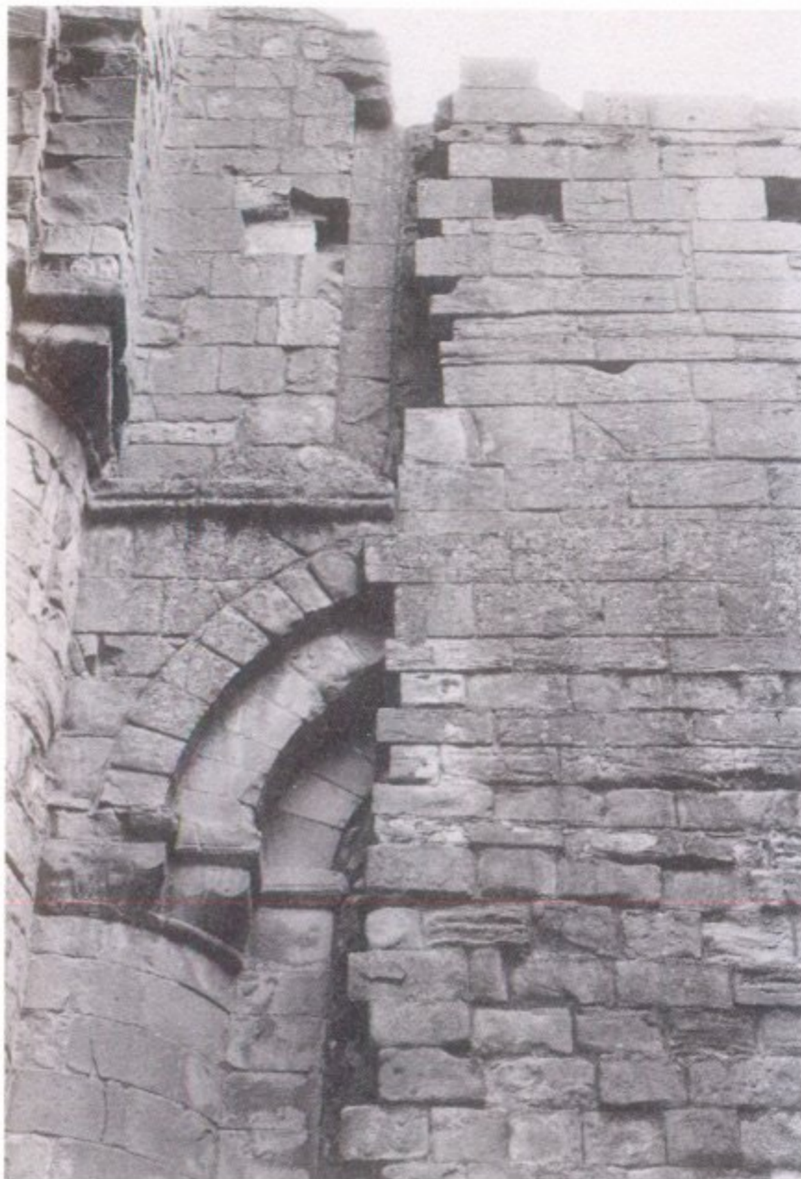
ILLUS 13 Jedburgh Abbey (interior): north transept, west gallery and clerestory
