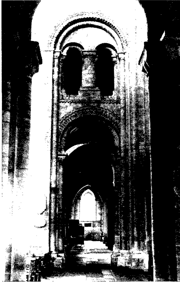
ILLUS 4 Romsey Abbey (Hampshire): south transept, elevation to south nave aisle and gallery
