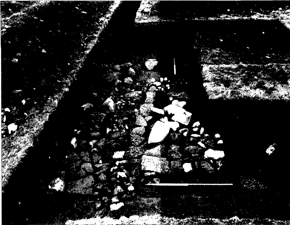
ILLUS 5 St Mary's Church, Bo'ness: stone base of Antonine Wall, seen from the south
