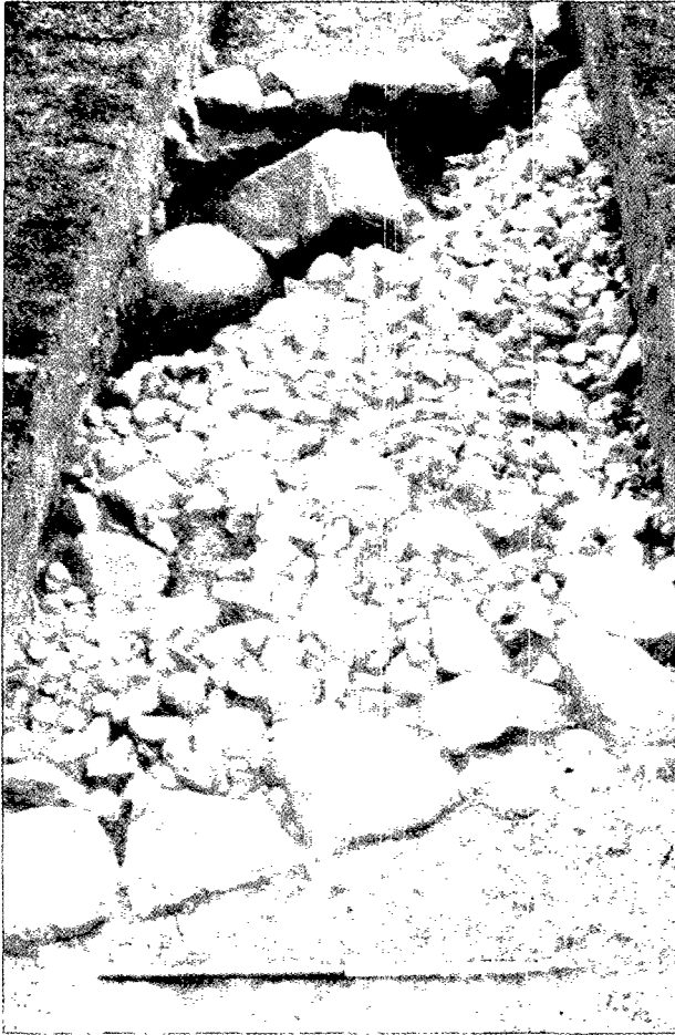
ILLUS 9 Beancross: the Wall base in trench A, looking north
