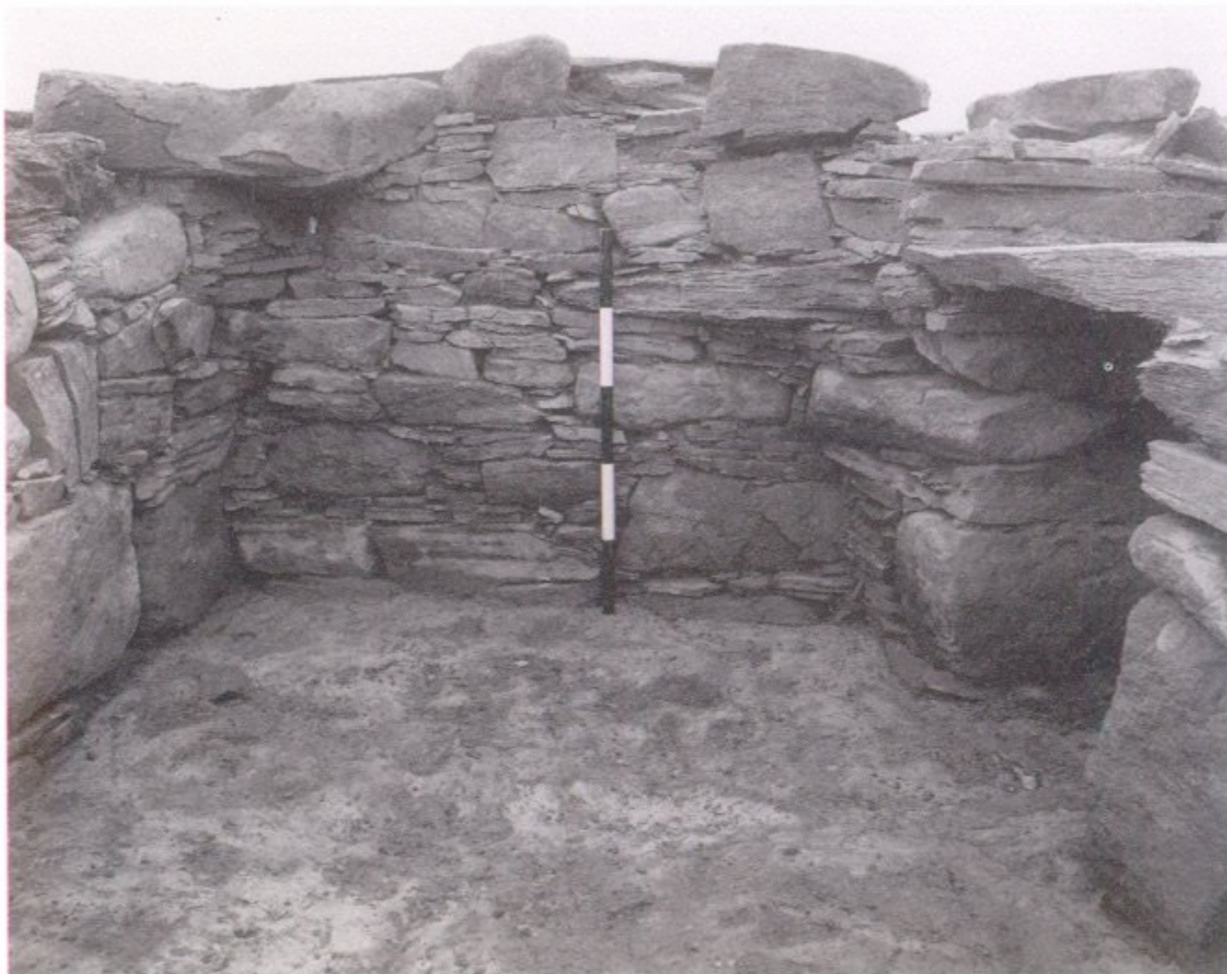
ILLUS 6 Scatness: east end of the blockhouse eastern cell showing the weight relieving structure over the entrance passage lintel
