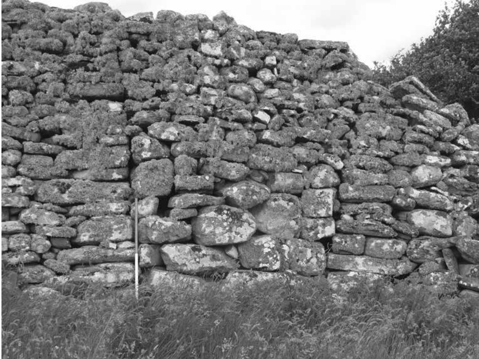
ILLUS 14 Photograph of Wall A with 'blocked-in' gap, from south
