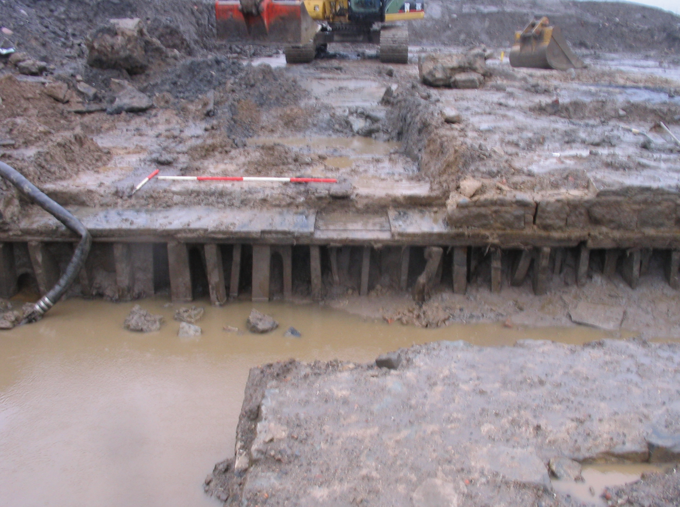
ILLUS 8 Elderslie House, Glasgow. Eastern Baltic pine felled in 1768 and 1774 was re-used as piling under one corner of this late 18th-century mansion
