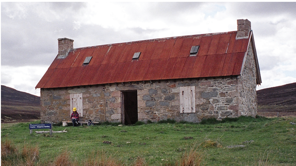
ILLUS 11 The Red House, on the Mar Lodge Estate. Pine felled locally in 1799 and 1808 was used to build a cruck-framed cottage, later converted into a keeper's lodge
