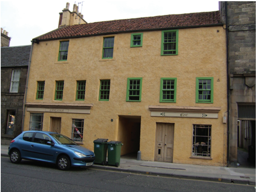
ILLUS 7 42–44 Market Street, Haddington. Eastern Baltic pine felled in 1765 and 1776 was used for the lintels, rafters and bressumer beams sampled during the renovation of this small townhouse
