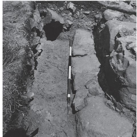
ILLUS 4 Photo of the south-west corner of the castle wall looking north, showing the stepped foundation (P–Q) of the tower
