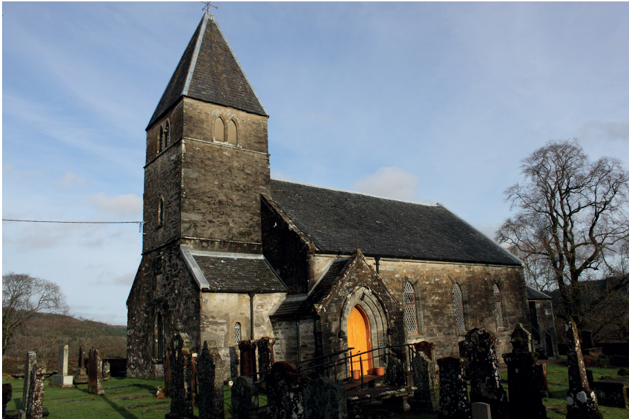
ILLUS 3 The parish church of Kilmichael Glassary, built in 1873 (photo: D H Caldwell)
