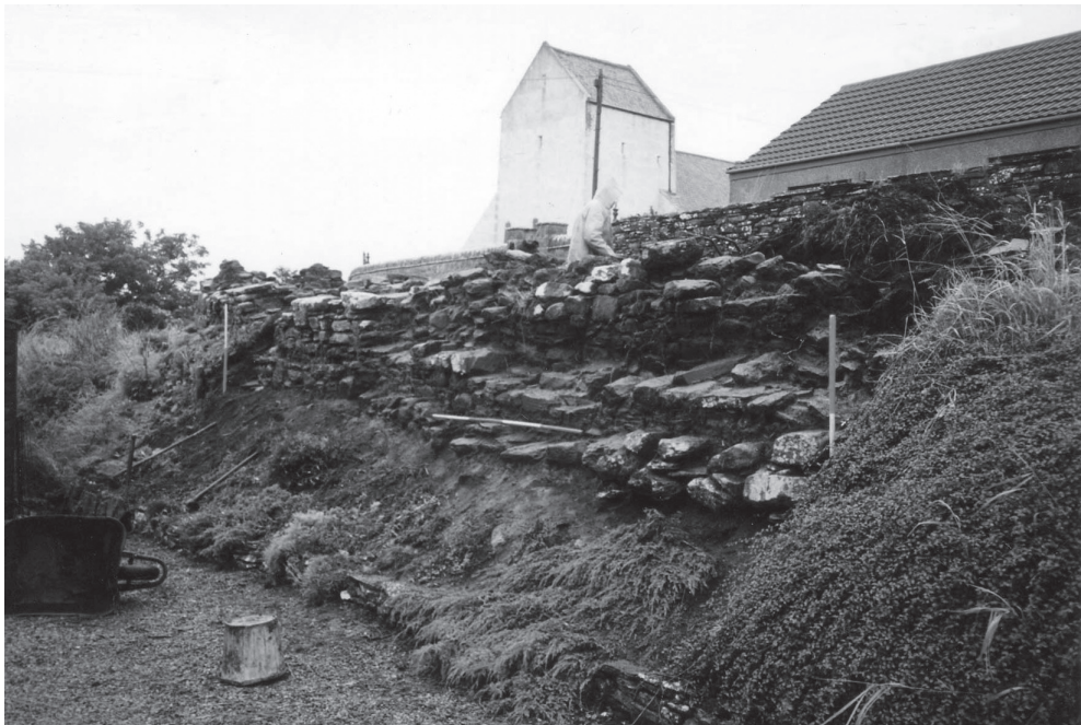
ILLUS 3 The site from the south-west, showing its location on the break of slope and the masonry exposed within the slope
