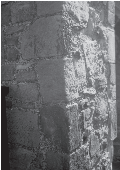
ILLUS 3 Stones in the north-west quoin of the Chapel of St Margaret at Edinburgh Castle are emplaced in Anglo-Saxon or Patterned style. Stones 7 to 11 are figured and in ascending order these are set BH, BVFL, BH, BVFR, BH. The oblique lighting displays the bedding in stone 8 the most clearly
