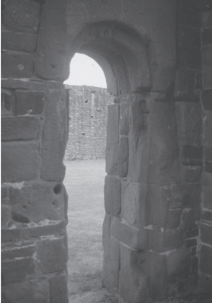
ILLUS 5 The interior (north side) of the tower door at Restenneth as illustrated in illus 4 . The west jamb, as the east, shows an absence of through stones and that the original structure was probably created from a thickness of three stones
