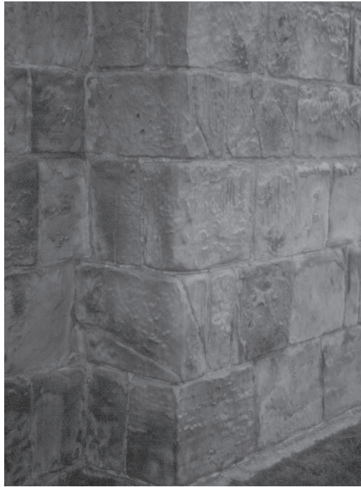
ILLUS 6 The detail of the plinth and stones 1 to 5 in the south-west chancel quoin of St Rule, St Andrews. Above the plinth the stones in ascending order are set with their bedding orientated, BH, BVFL, BVFR, BVFL, BVFR, in Anglo-Saxon or Patterned style
