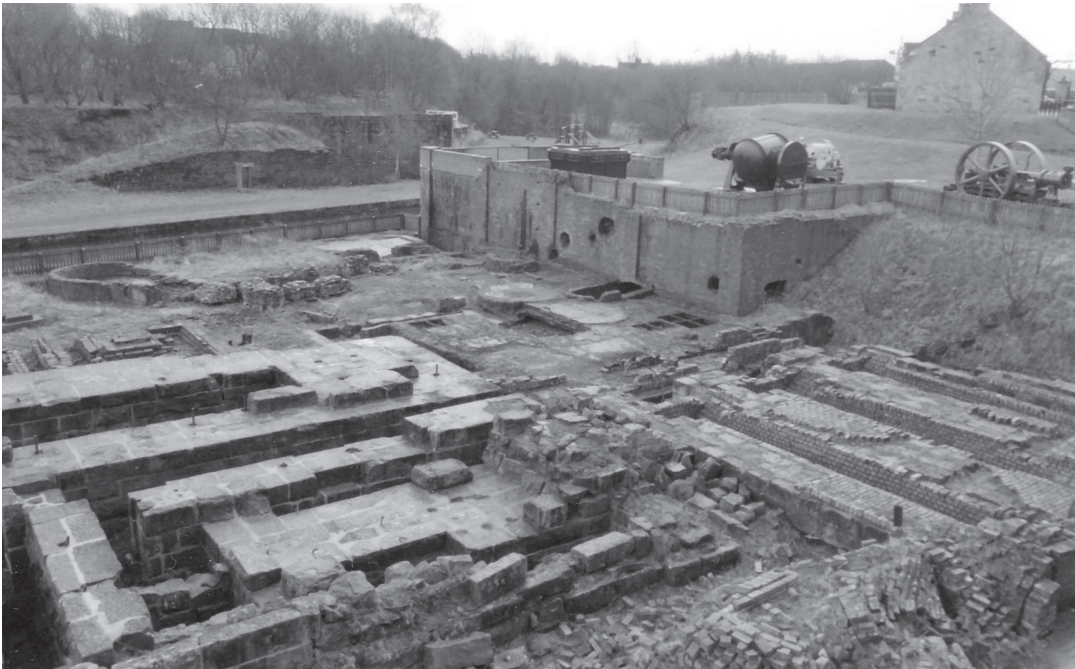
ILLUS 11 View, from the north, of the south-west corner of the site in 2004, showing the bases of the Lancashire boilers on the right of the frame, the engine house in the foreground and the chemical recovery plant behind. The Gartsherrie Cut (a branch of the Monkland Canal) lies beyond the chemical plant
