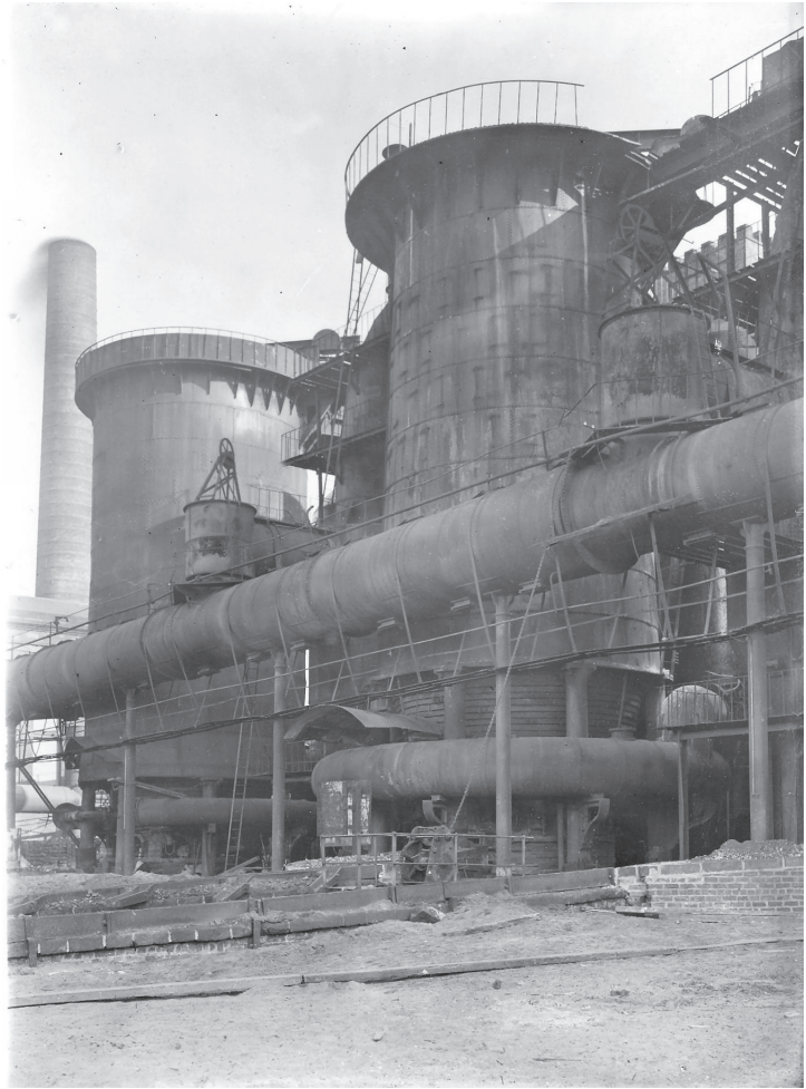
ILLUS 18 View of some of the furnaces at Glengarnock, Ayrshire in the late 19th century (note the hot blast horseshoe main encircling one of the furnaces and the large exhaust gas pipe at a higher level)
