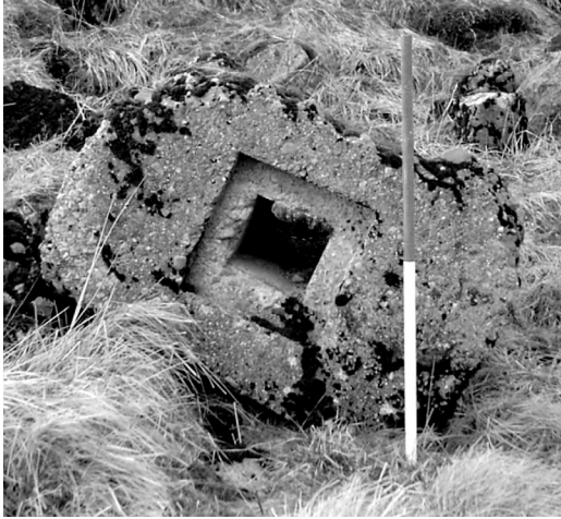
ILLUS 8 One of the probable roadblock sockets, now lying below the modern road at the Devil's Elbow
