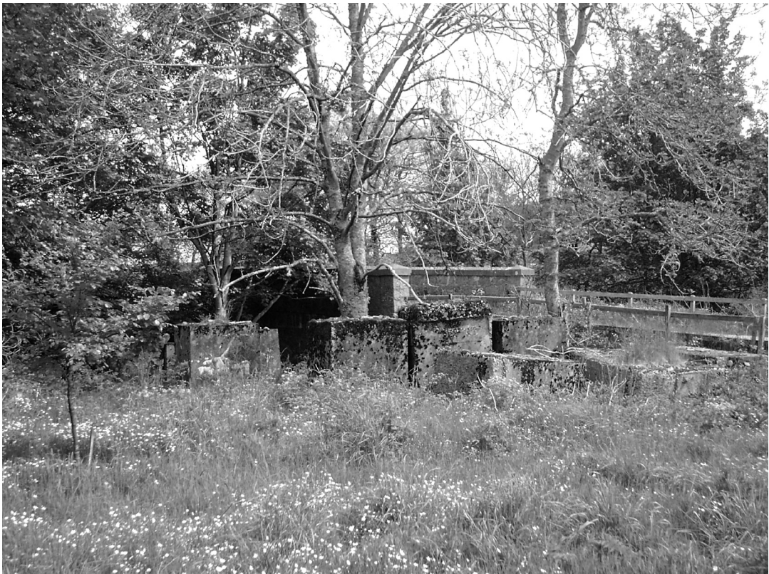
ILLUS 14 Haugh Head Bridge showing cubes
