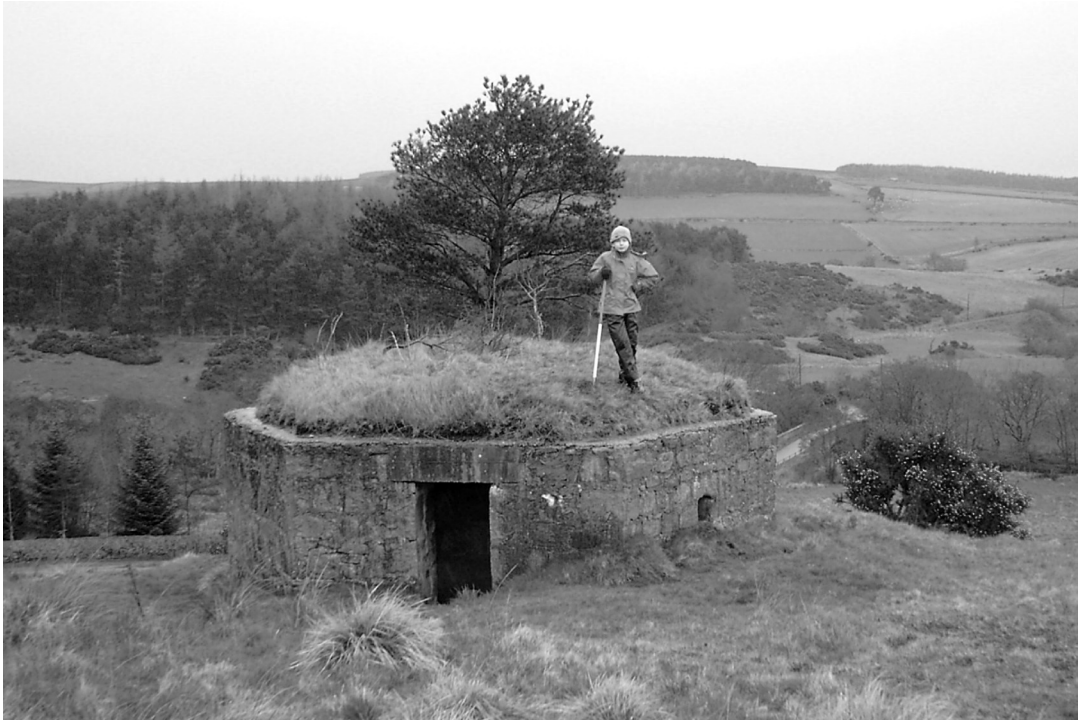
ILLUS 15 Haugh Head south pillbox from the south; the bridge is visible immediately to the right of the pillbox
