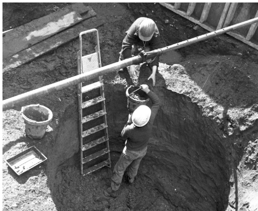
ILLUS 7 Canal Street I. A large quarry/rubbish pit
