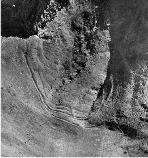
ILLUS 4 Aerial view of Kaimes Hill in 1964: west lies at the top of the photograph ( Photograph by Planair: Crown Copyright )
