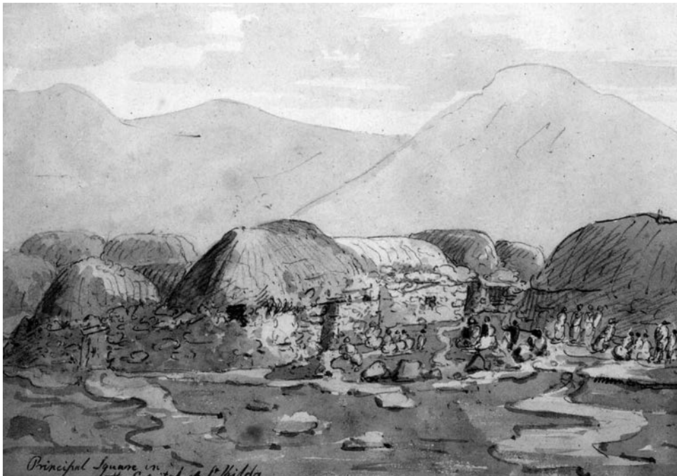
ILLUS 7 Acland's illustration of the 'Principal Square' (1812) for comparison with illus 6 ( National Trust )
