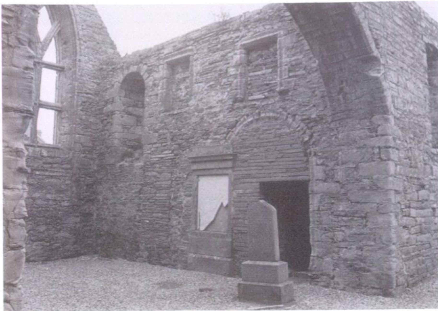
ILLUS 10 Old St Peter's: west wall of south aisle from the nave (G Watson)
