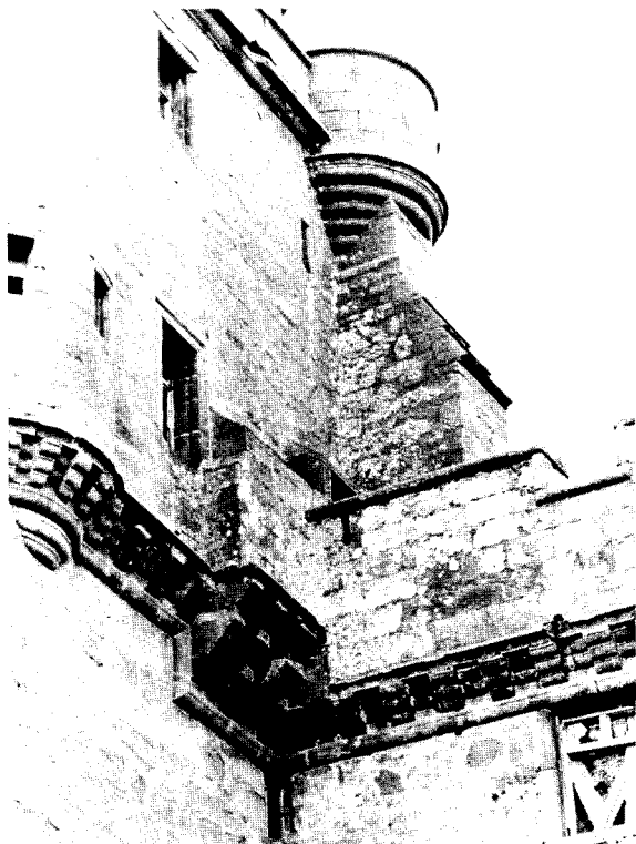
ILLUS 13 Re-entrant angle at parapet level, showing machicolation over entrance and flanking shot-hole
