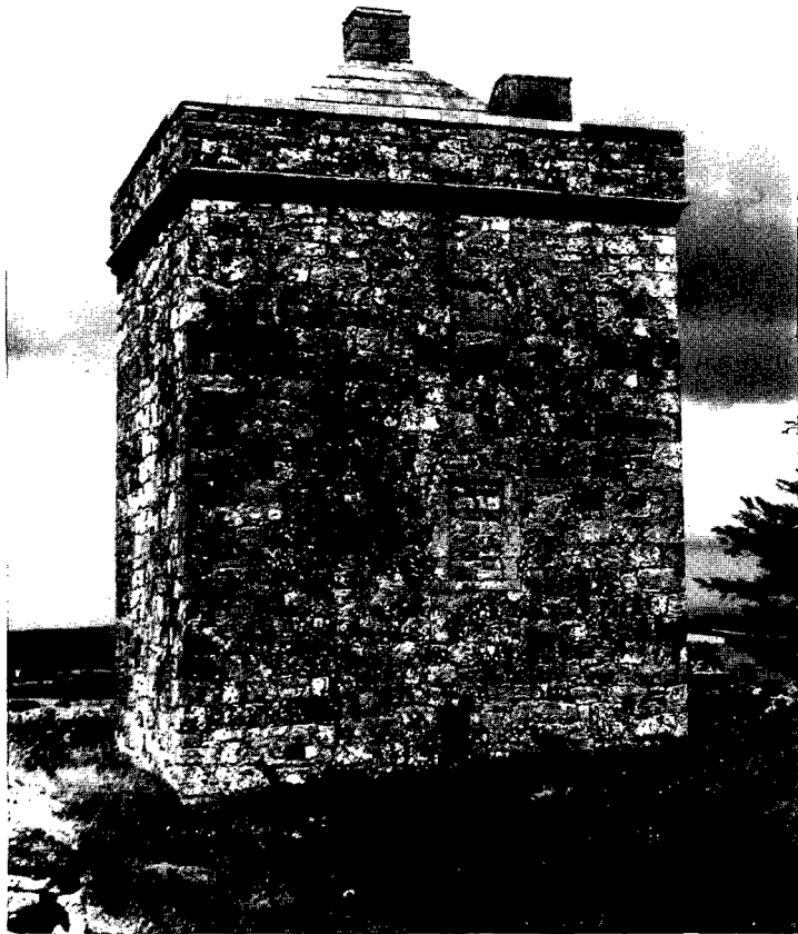
ILLUS 20 Repentance tower from the south
