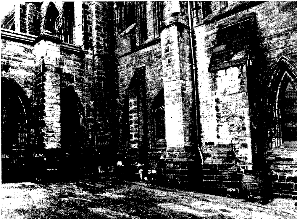
ILLUS 2 The junction of the Blackadder Aisle (on the left) and the choir crypt
