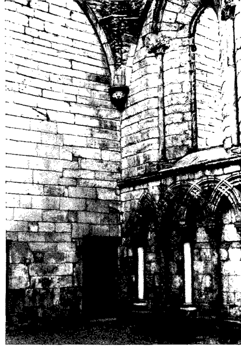
ILLUS 2 Holyrood Abbey: interior, junction of north aisle wall (right) and east wall of tower (left) (photo: author)
