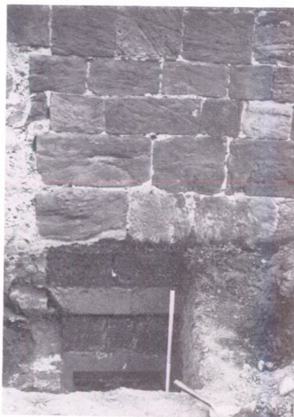
c Buttress and chamfering on NE corner of the tower
