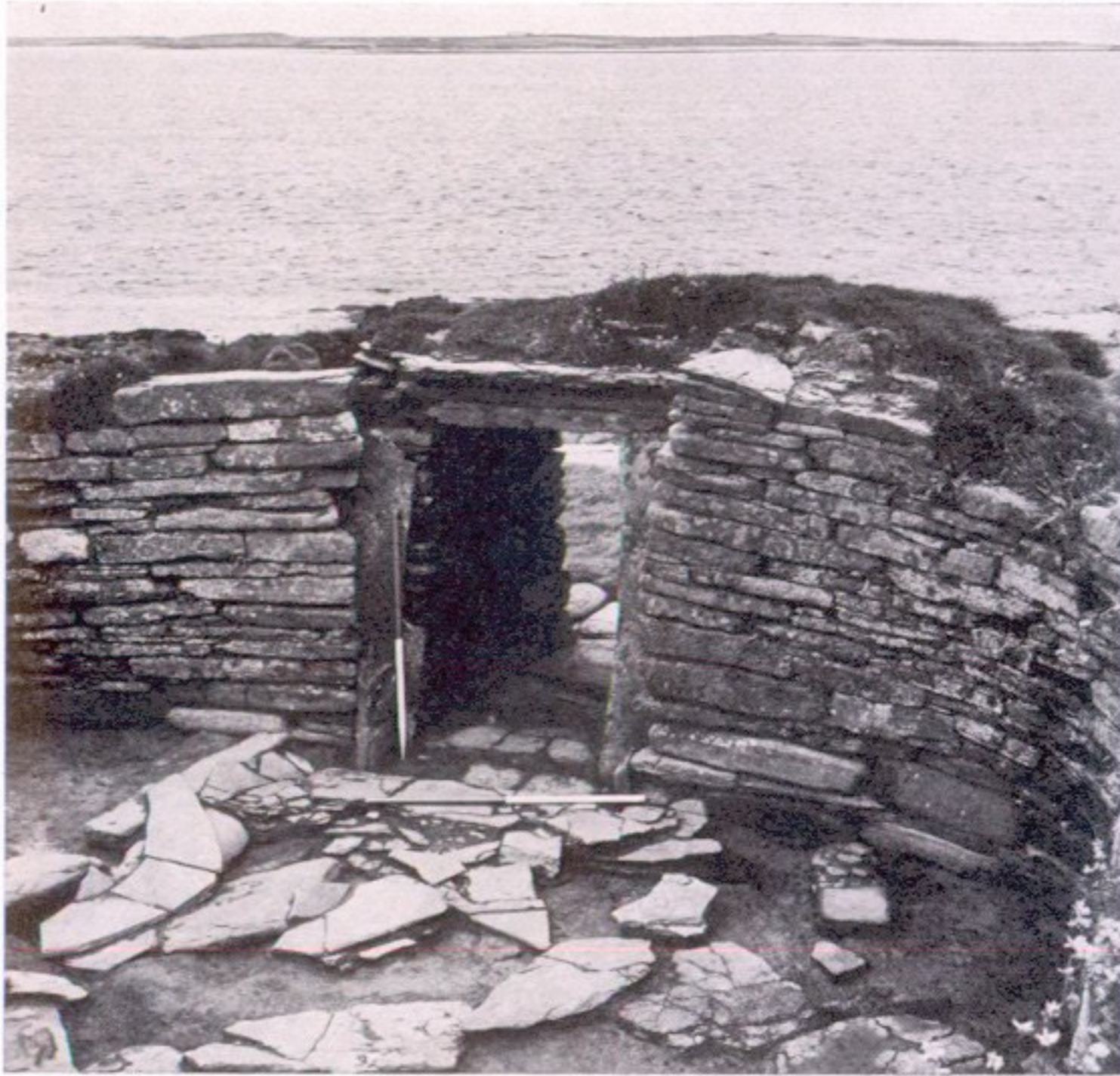
a Inner end of entrance passage, house 1
