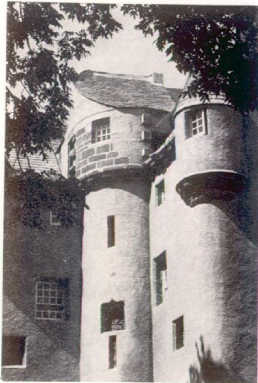
b Stair tower and Cap house: after restoration
