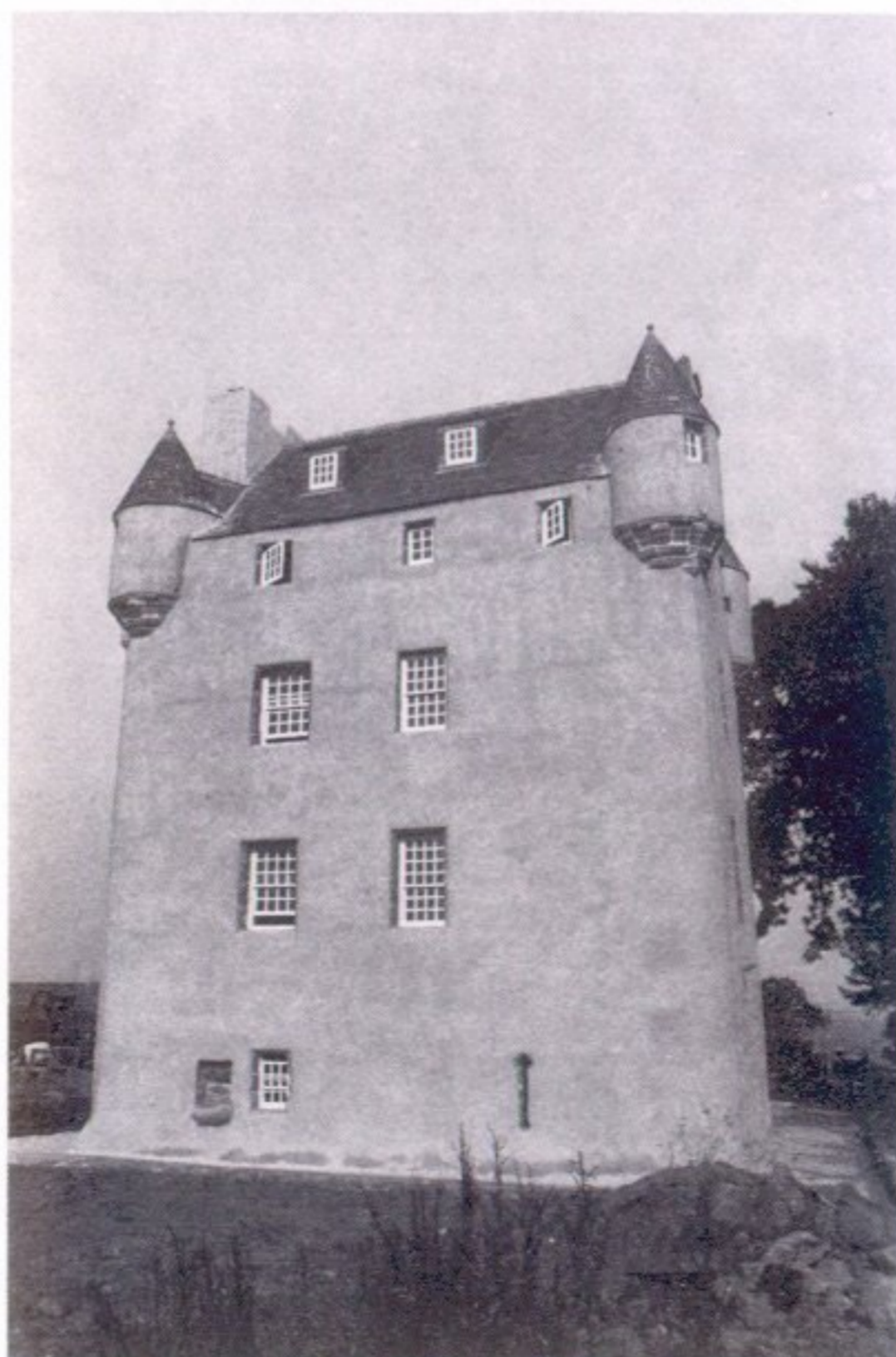
b West front: after restoration
