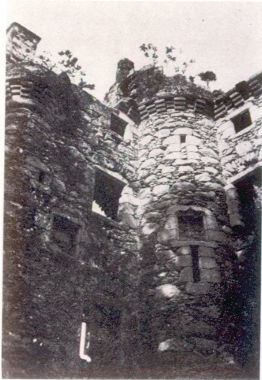
a Stair tower and Cap house: before restoration
