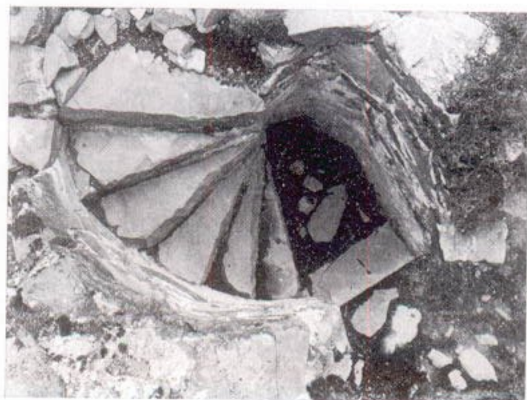
c North Tower, stair well
