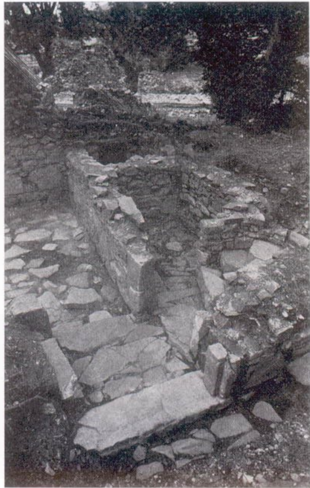
b South Tower entrance and mural chambers with N Tower beyond
