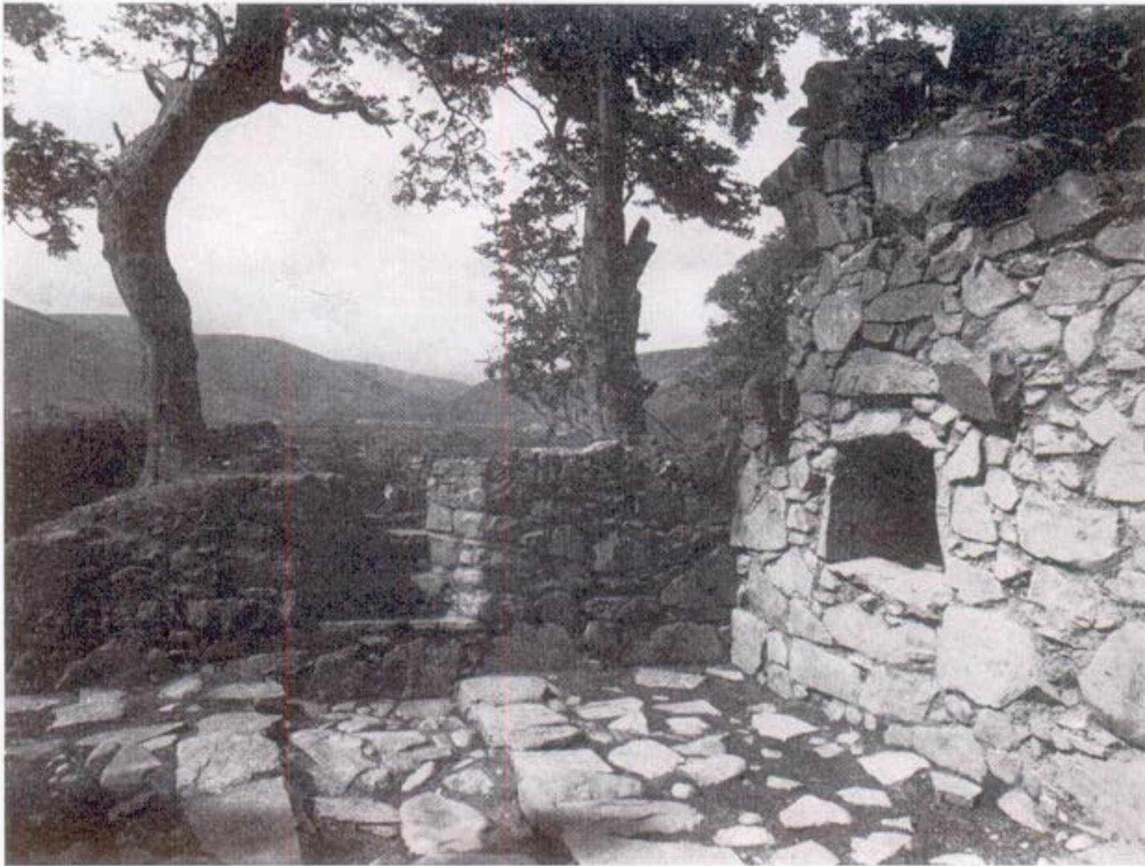
a South Tower, NW corner of basement showing corbels for entresol floor and start of vault
