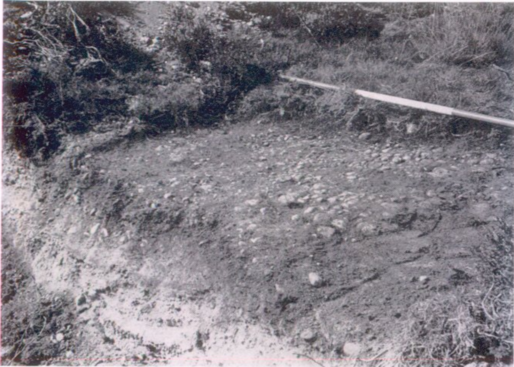
a Typical gravel running surface on the Wade Road, recently exposed
