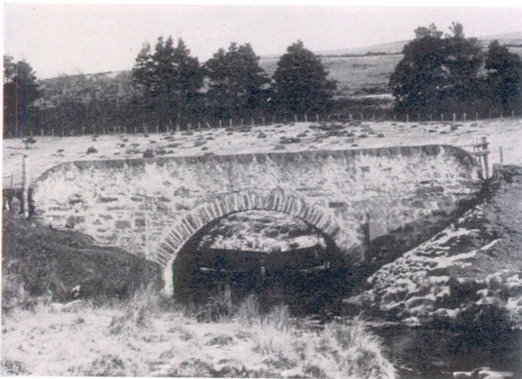
b A Parliamentary Bridge, Type 3: Bridge over the Allt Cosach, Drumbain
