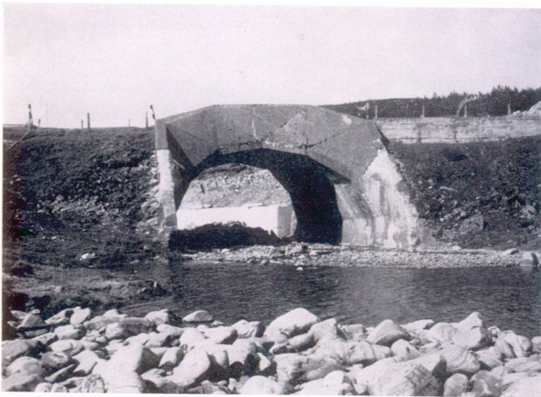
b A concrete arch with 6 facets carrying the A9 over the Edendon Water
