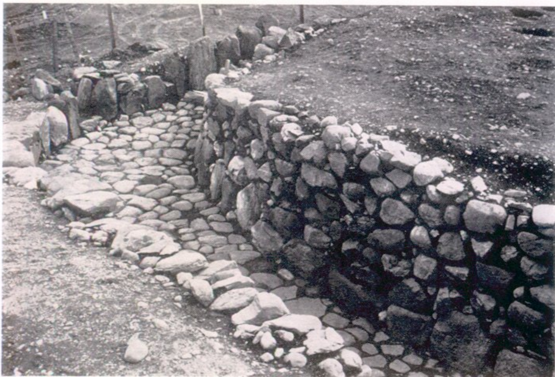
b Terminal of souterrain chamber
