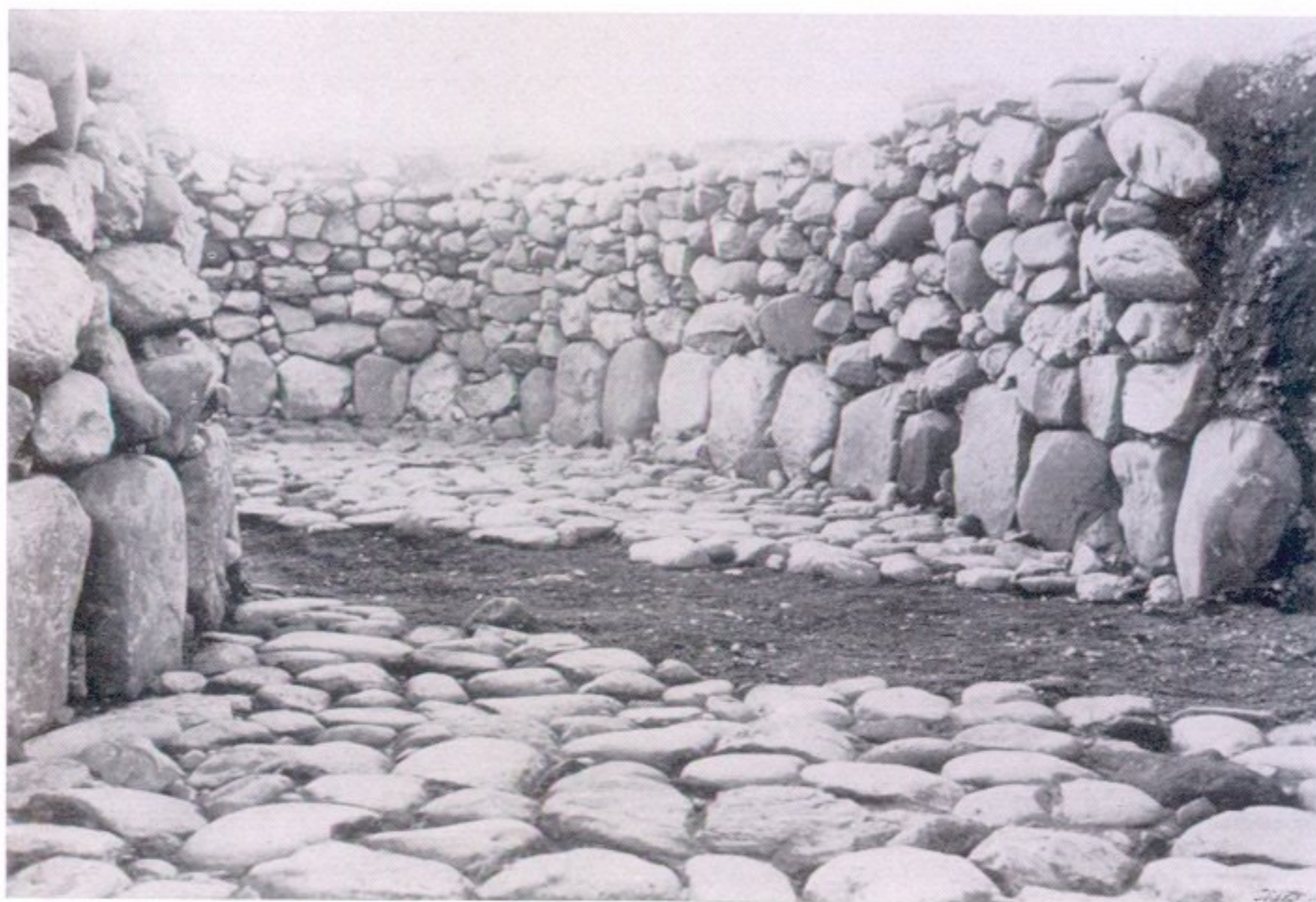
b Floor level view into terminal from mid-chamber
