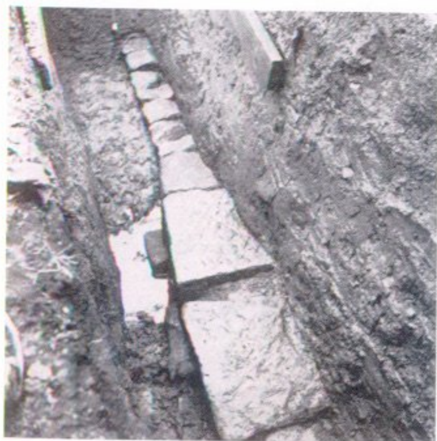
Mouth of culvert through the S rampart
