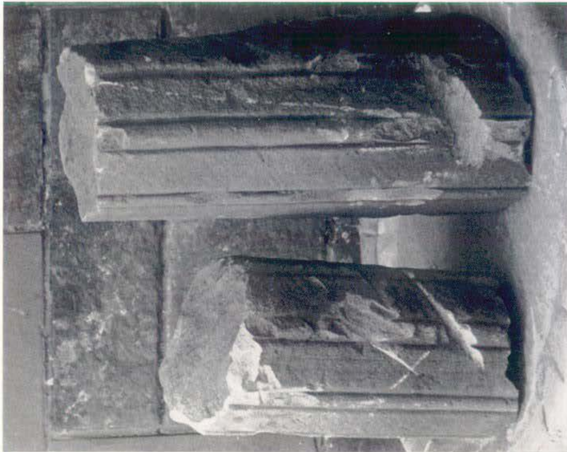
a Stones no. 7, shafts A & B
