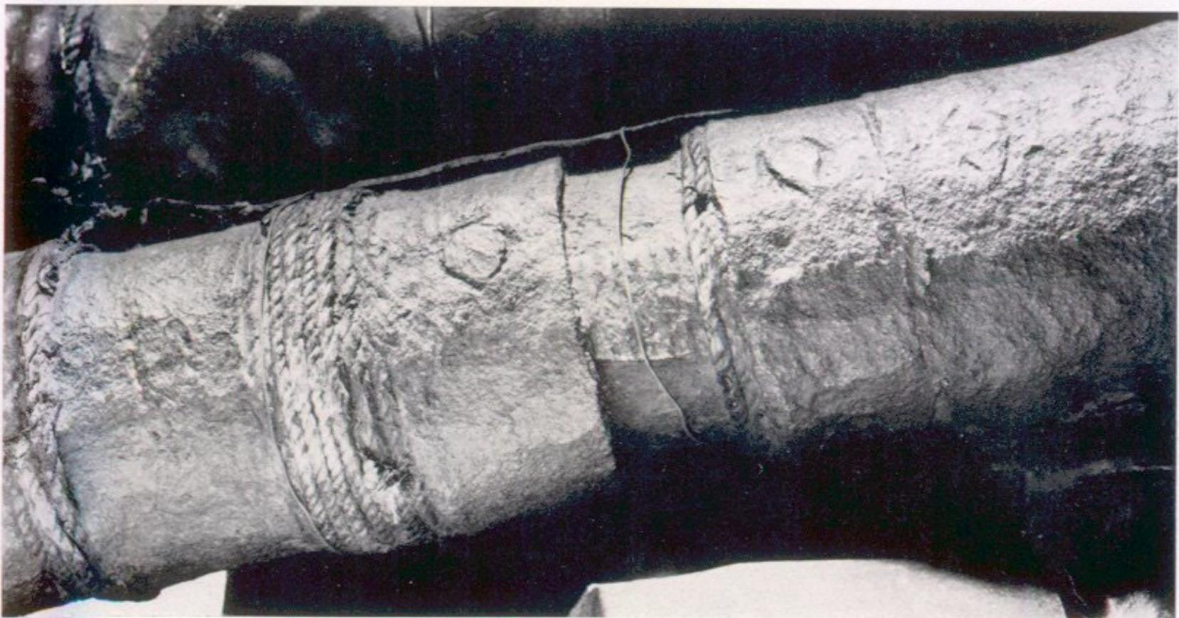
c Detail of barrel construction showing rivets and copper plate covering barrel seam
