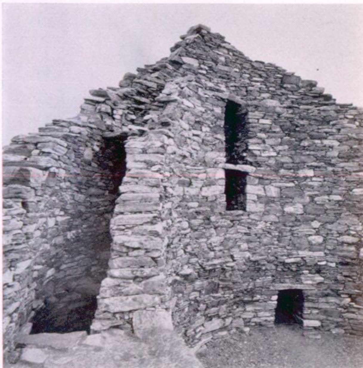
b Partial view of interior from N, chamber A on left
