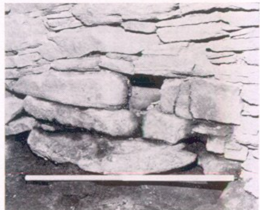
c Interior of chamber A, showing void (2) in outer wall
