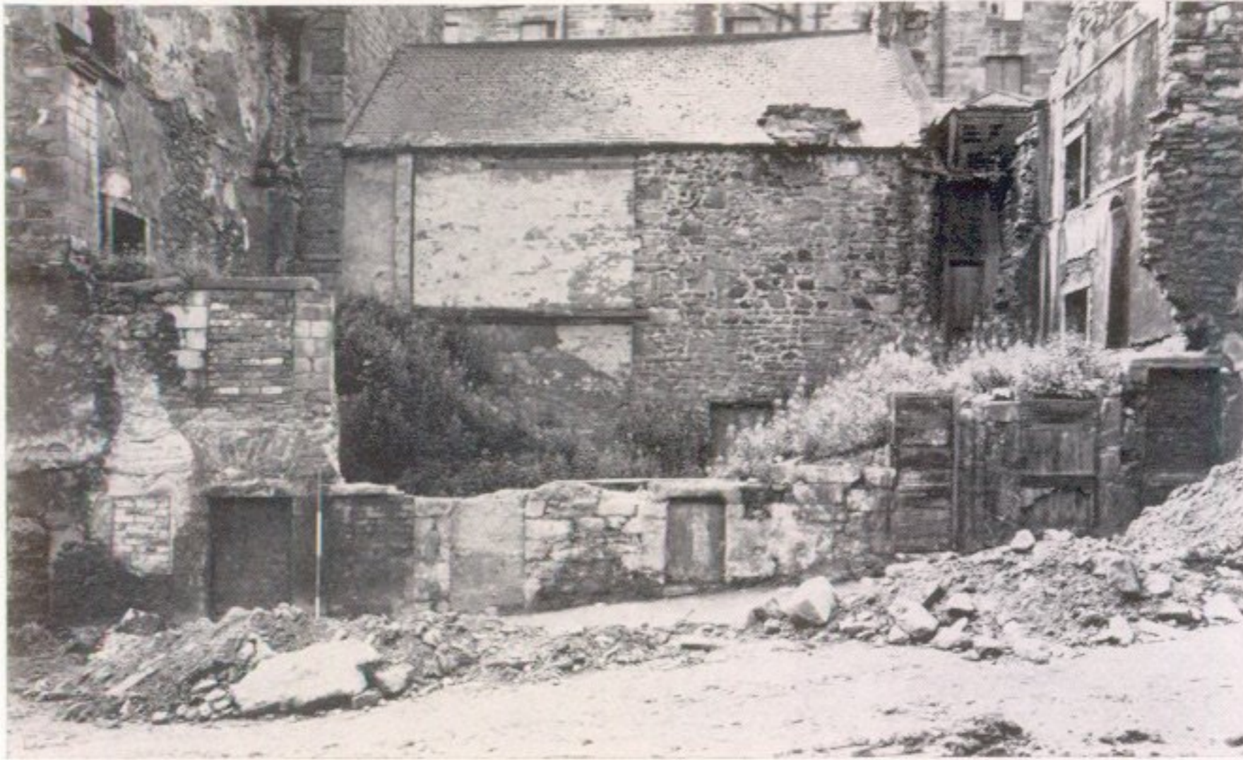
a Front of Area 3 house before excavation
