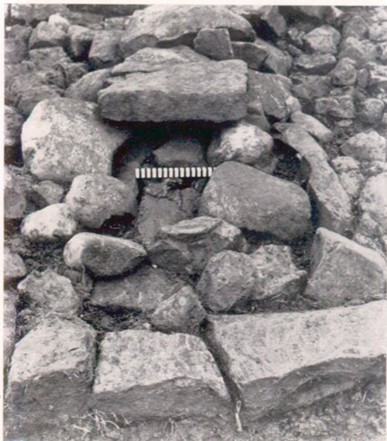
b Bantaskin: repaired N kerb blocking mouth of culvert
