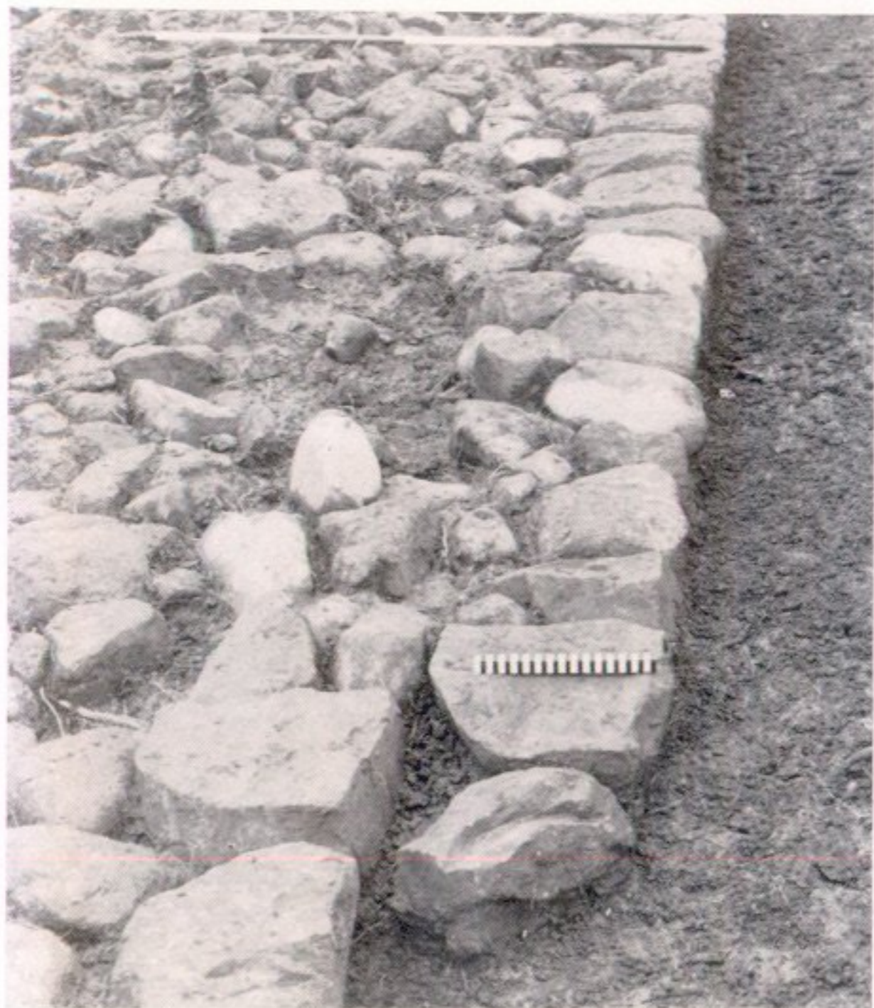
a Bantaskin: repair to N kerb of stone base
