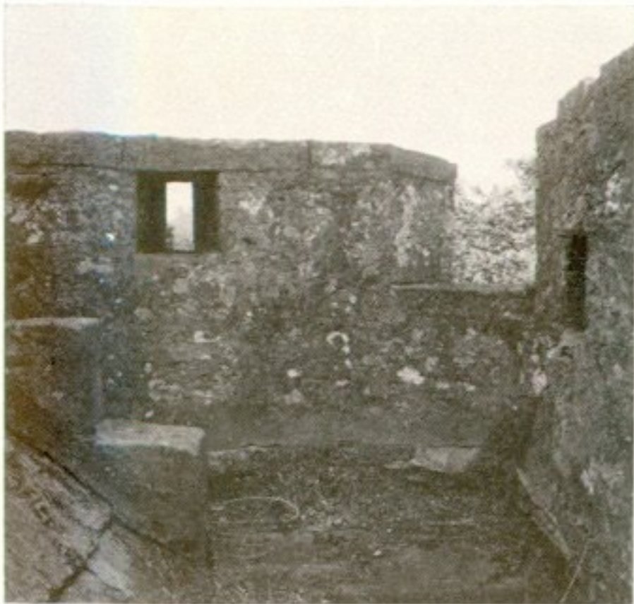
a Hoddom: NE corner round on parapet walk with protected shot-holes on either side of open embrasure (later sixteenth century)
