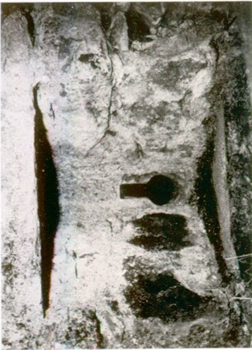
a Newark: miniature inverted key-hole shot-hole in S flanking tower of curtain wall, from inside (mid sixteenth century)
