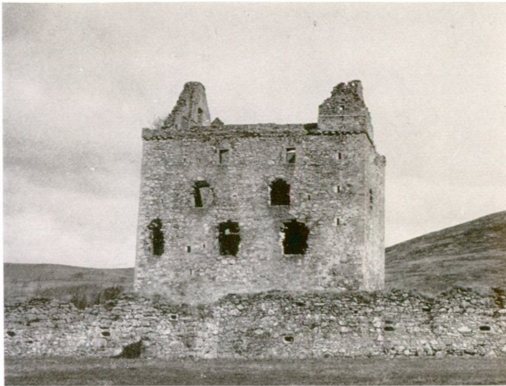
a Newark Castle from the S, showing shot-holes in curtain wall (fifteenth century) and S flanking tower (mid sixteenth century)
