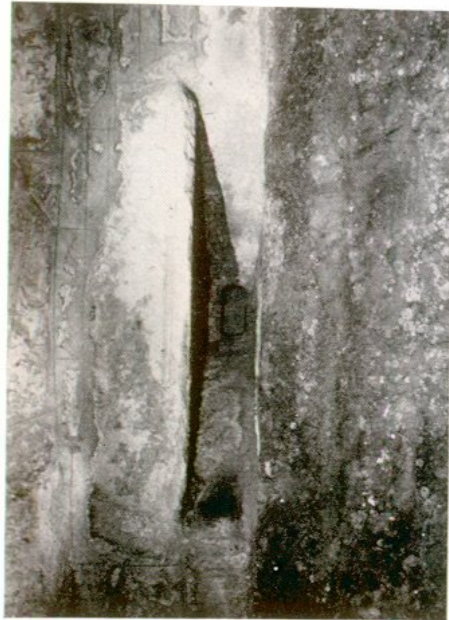
c Bonshaw: rectangular splayed shot-hole, S basement (third quarter sixteenth century)
