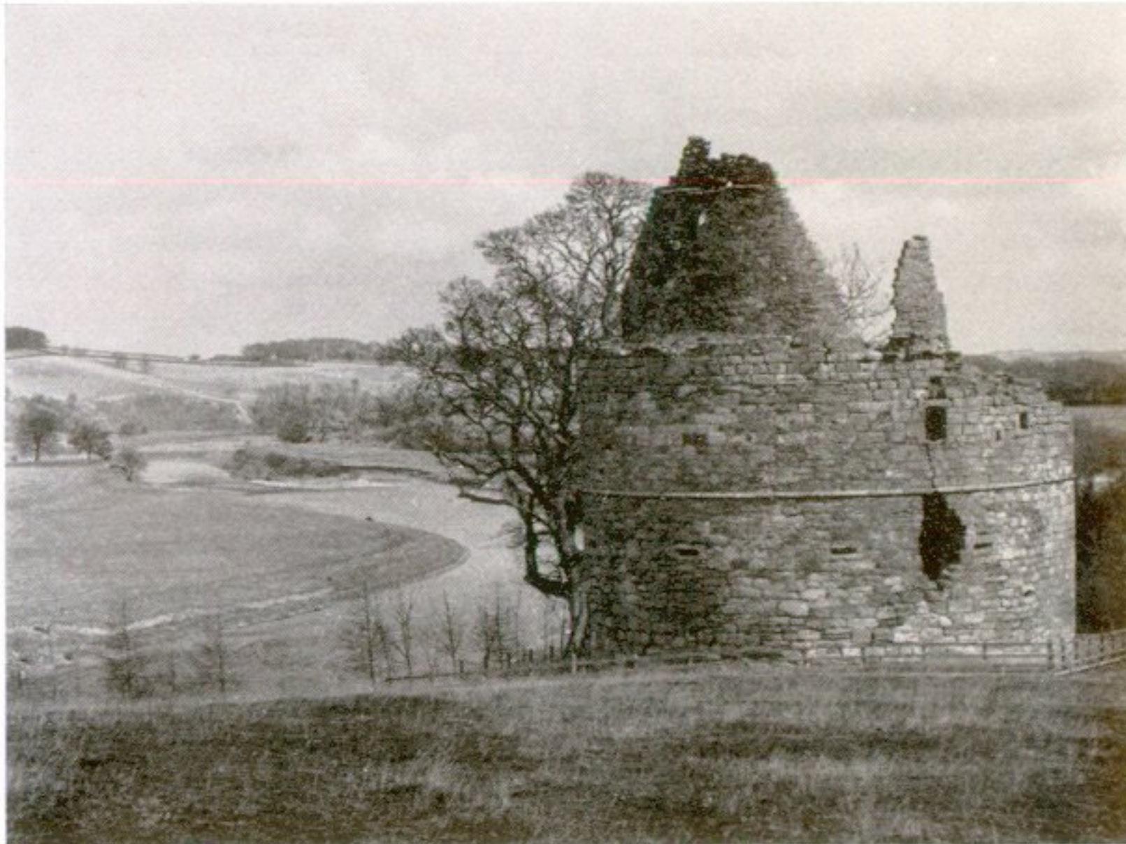
b Littledean Tower: lower level shot-holes obscured by rising ground
