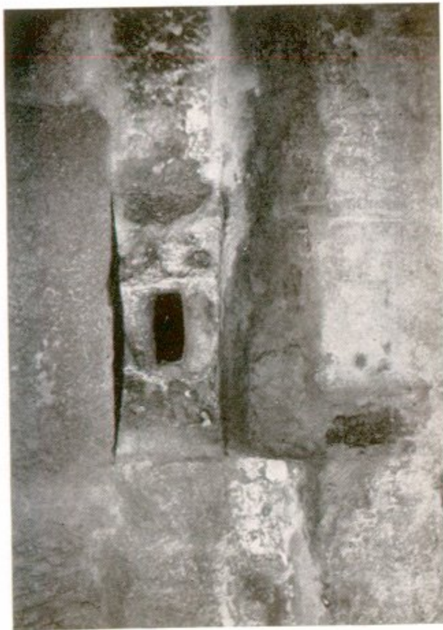
a Bonshaw: guard's shot-hole at entrance, from outside (third quarter sixteenth century)
