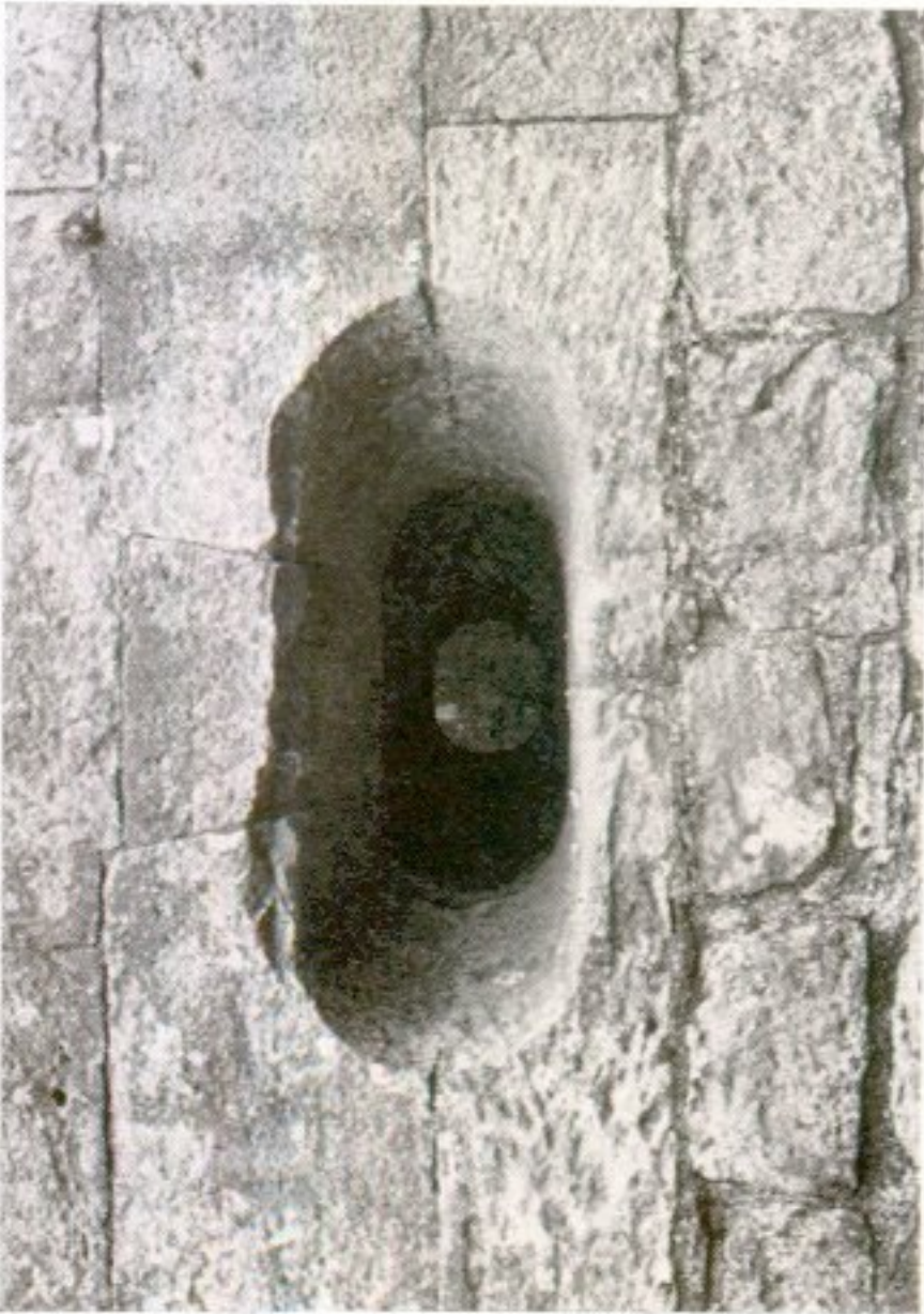
a Hermitage: oval splayed shot-hole inserted in old W entrance doorway, seen from outside (1540)
