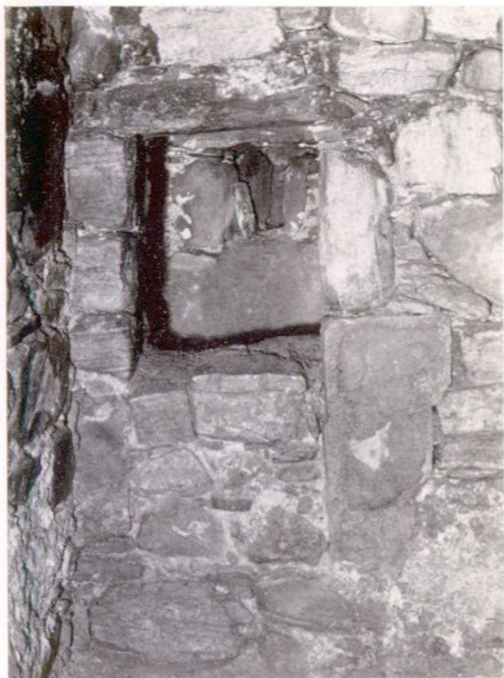
a Ground-floor doorway to mural staircase in S wall of tower-house
