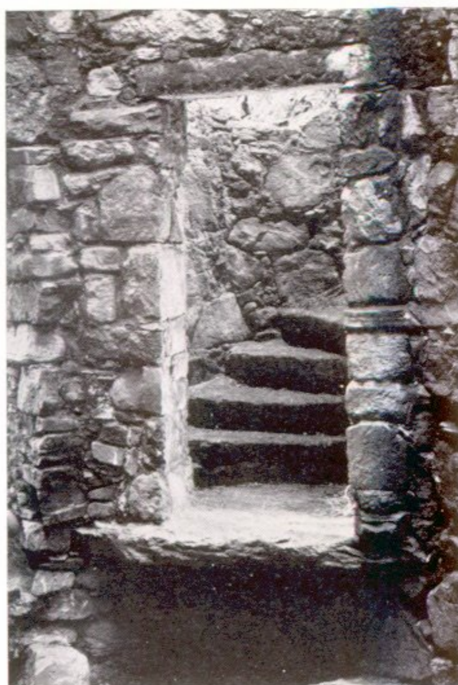
b First-floor doorway to turnpike-staircase in S wall of tower-house
