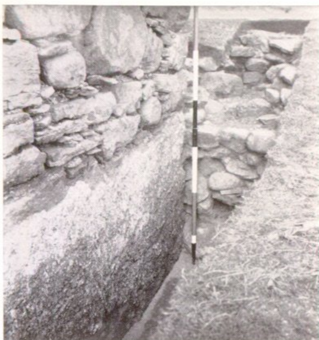
a Trench across battery, showing harling of tower-house wall preserved beneath soil-level, and clay-bound rear of battery-wall
