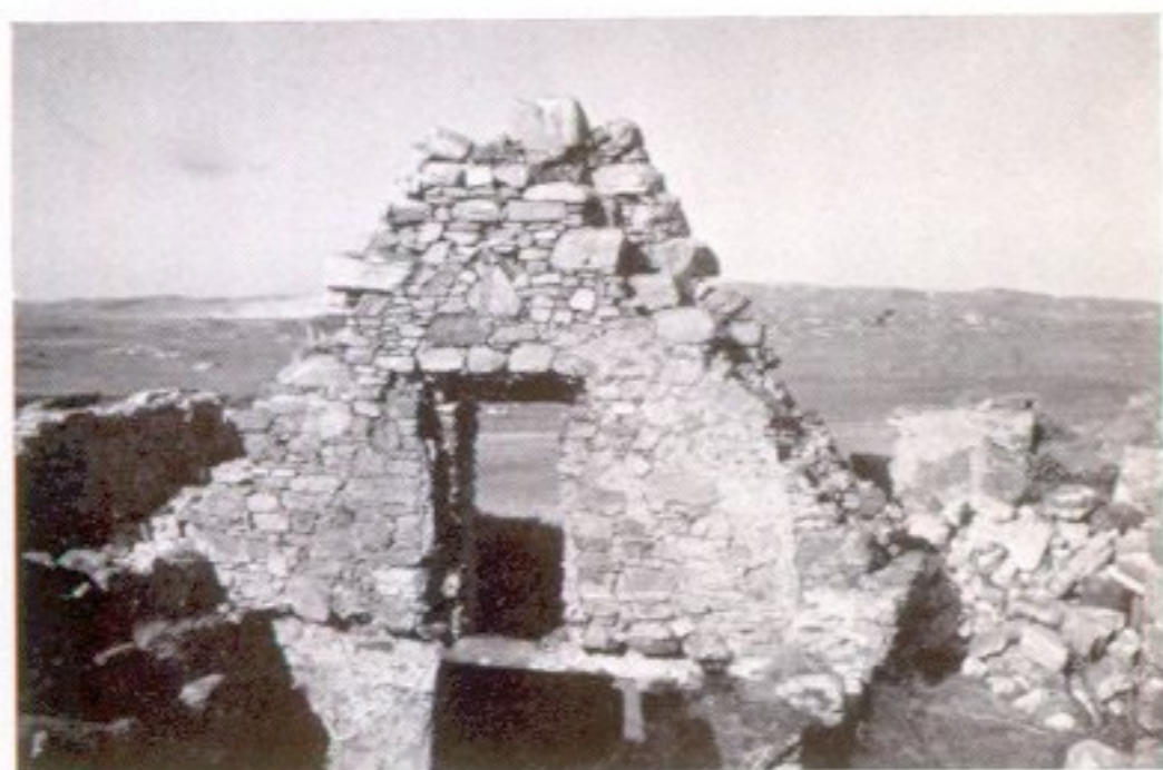
c Gable-wall of tower-house showing outline of earlier gable-head
